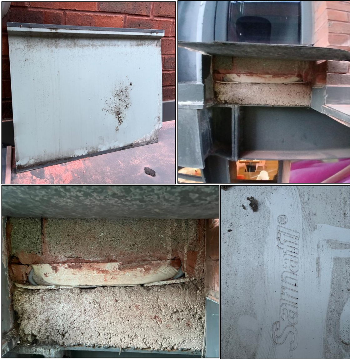
Figure 22 – Typical inspection images for EWT3 taken by Octa Fire.
