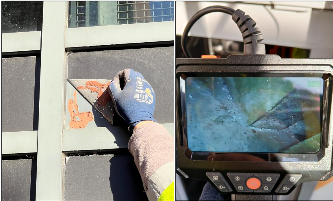
Figure 28 – Typical inspection images for EWT5 taken by Octa Fire.
