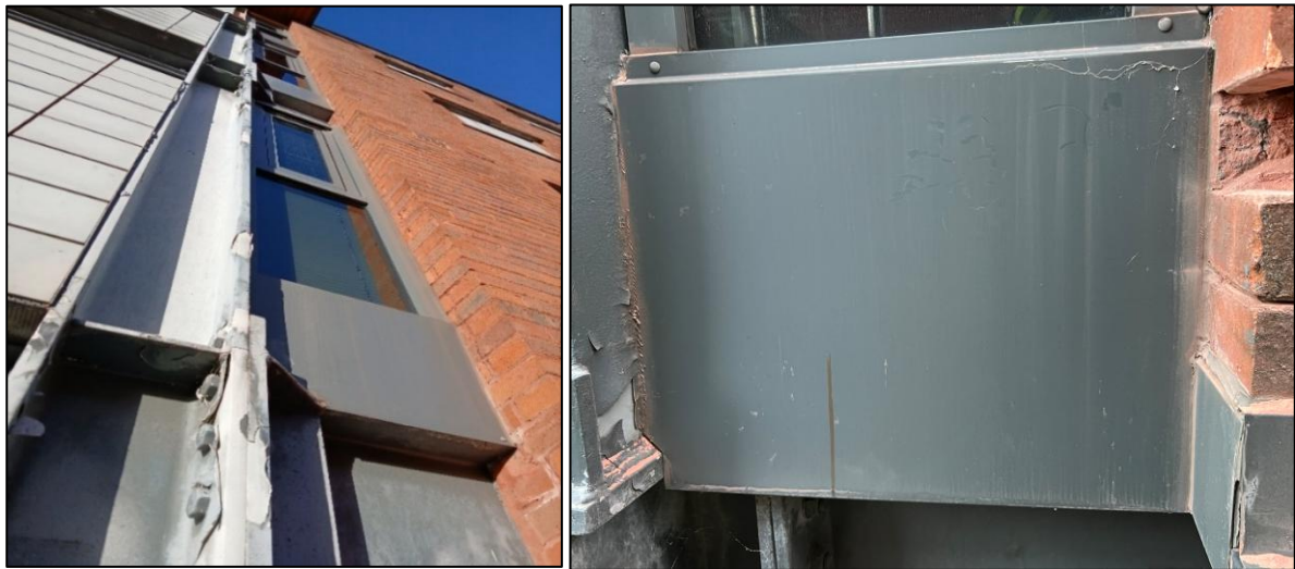
Figure 14 – Grey metal cladding panels – EWT3.
