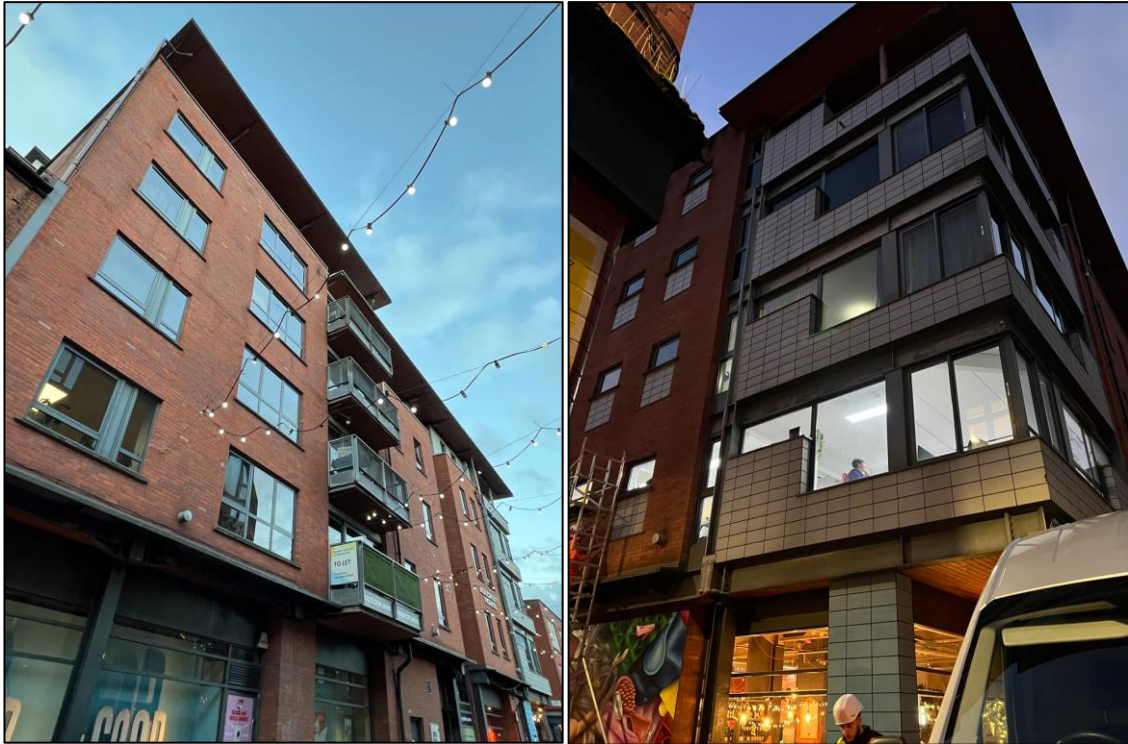
Figure 1 – Typical building images of Agecroft House taken by Octa Fire during our site visit of the building.
