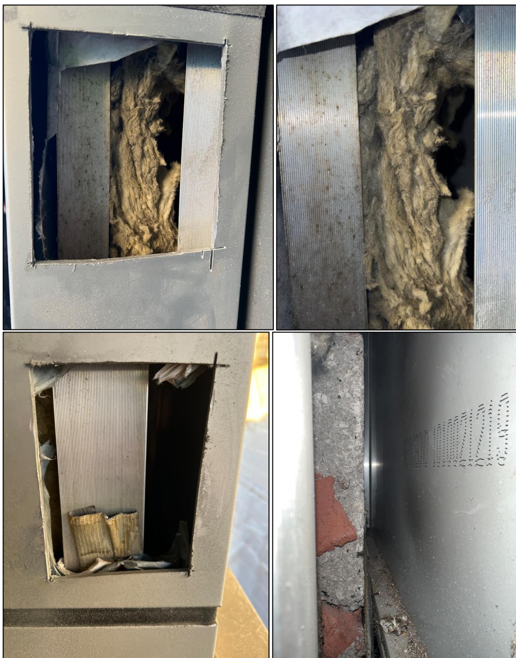
Figure 25 – Typical inspection images for EWT4 taken by Octa Fire.
