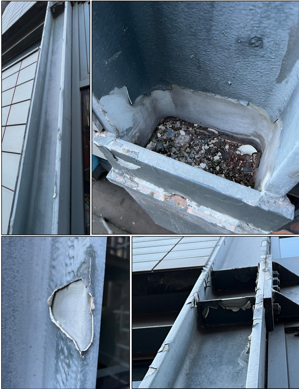
Figure 23 – Typical inspection images of steel structure taken by Octa Fire.
