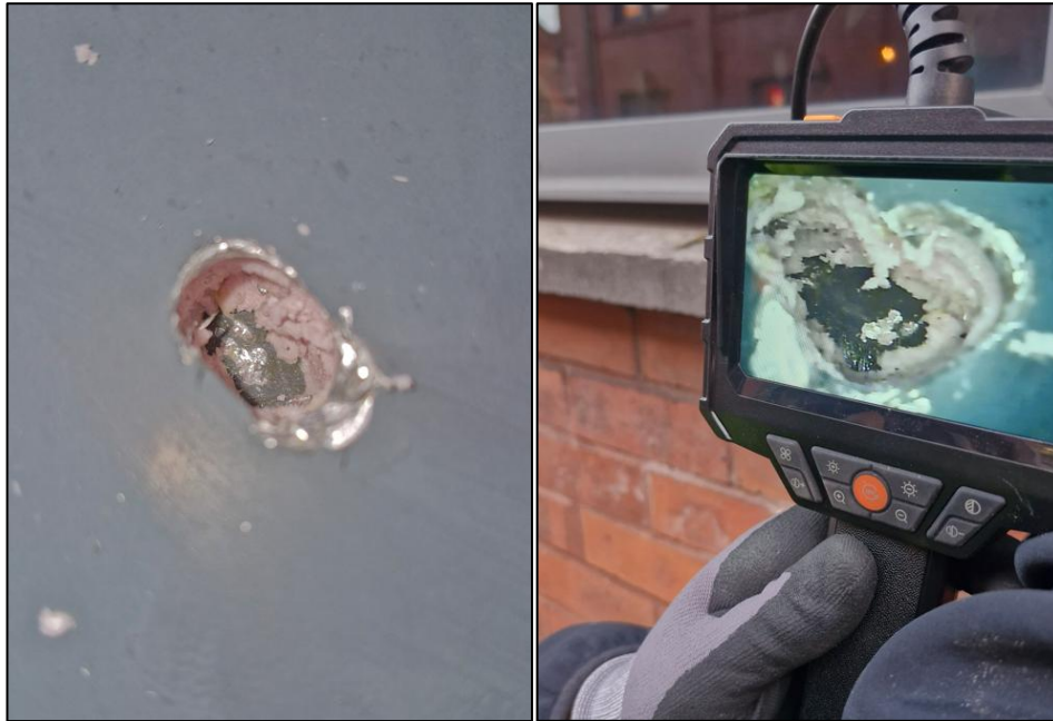
Figure 27 – Typical inspection images for EWT5 taken by Octa Fire.
