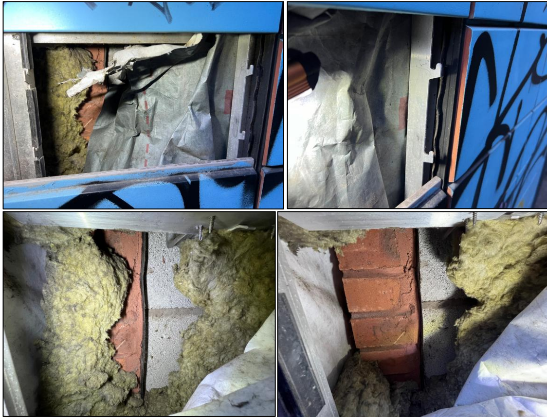
Figure 20 – Typical inspection images for EWT2 taken by Octa Fire.
