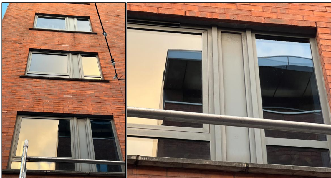
Figure 16 – Grey insulated window cladding panels – EWT5
