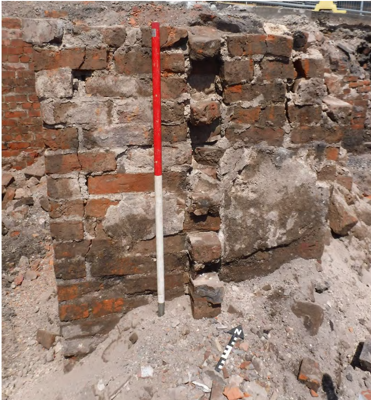
Figure 5. Wall {022} flanked to the left by buttress {016} and to the right by buttress {033}, looking northwest, 1m scale.
