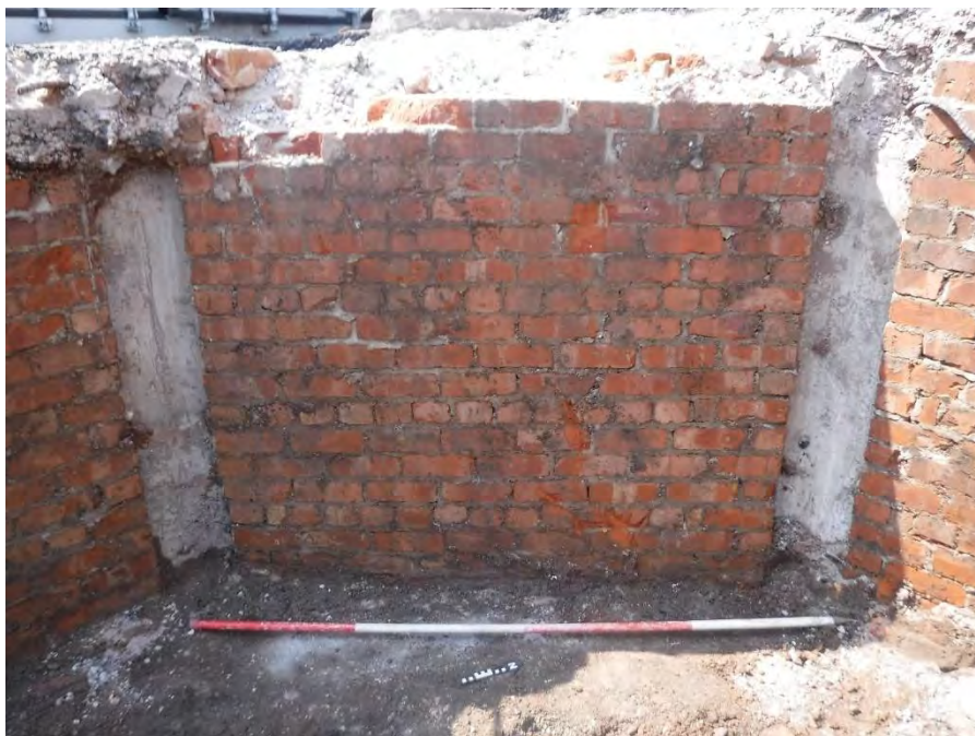
Figure 23. Wall {013}, a trapezoidal structure forming the northwestern corner of the mid-20 th Century structure, looking northwest, scale 1m.
