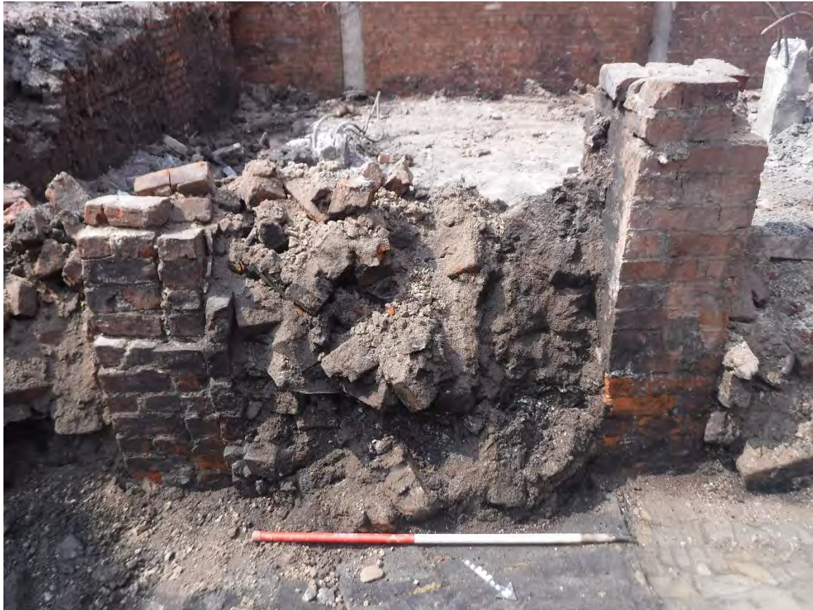
Figure 13. Collapsed fireplace uncovered in House F, comprising buttresses {041} and {040} (left to right), looking southwest, scale 1m.
