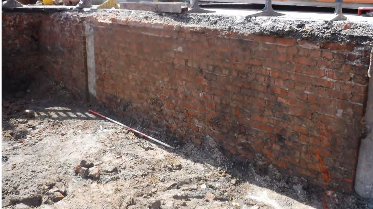
Figure 21. Walls {023} and {024}, two 20th century walls separated by concrete pillars alike to stanchions {213} {214} and {223}, looking southwest, scale 2m.
