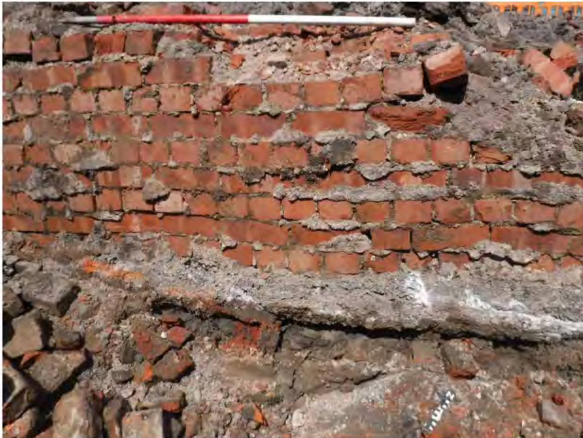
Figure 28. Wall {215} a heavily truncated wall possibly acting as a party wall for the southeastern section of mid-20 th -century warehouse, scale 1m.
