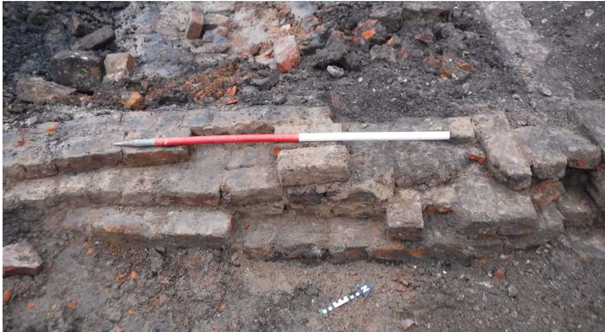
Figure 18. Wall Foundation {230}, looking west, scale 1m.
