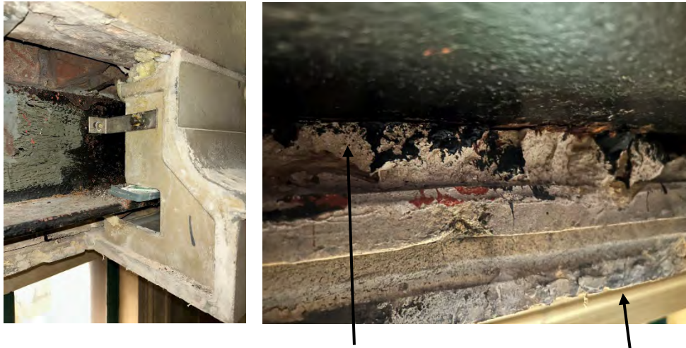
Underside of structural steelwork
