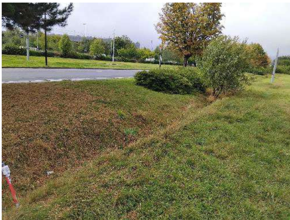
Plate 8. View looking south-west towards Aviator Way showing the drain within the southern side of the study site
