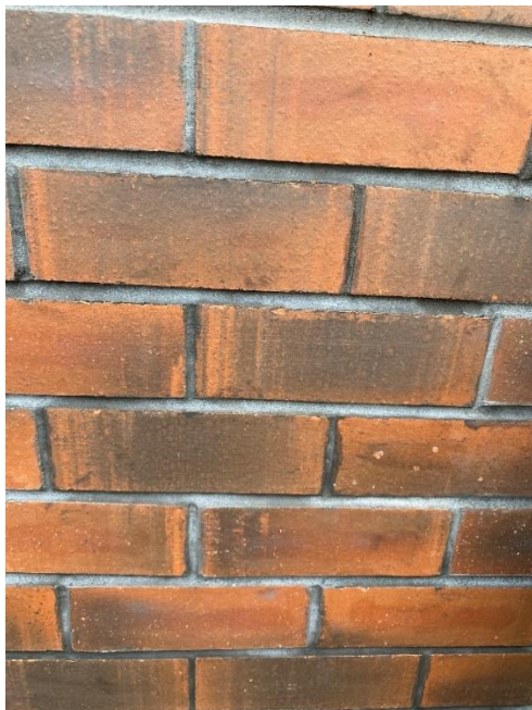
Figure 7: Mortar in situ with brick 19.09.26
