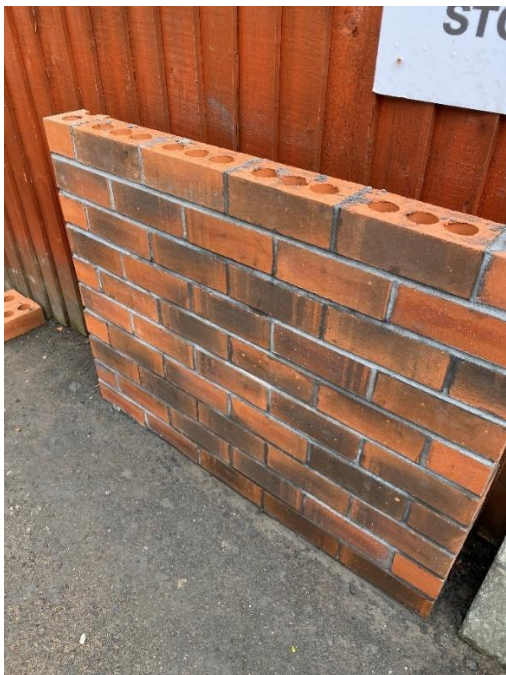
Figure 2: On site brick sample 19.09.26
