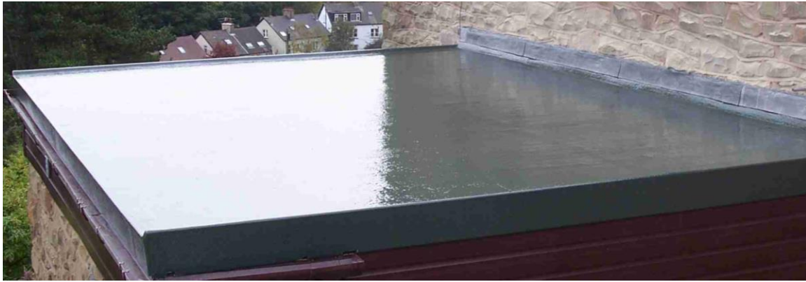
Figure 20: Flat Roofing system
