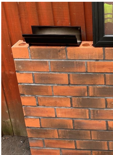
Figure 10: Sample on site with brick sample
