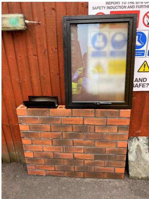
Figure 14: Window on site with brickwork and Guttering 19.09.26
