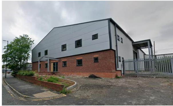
Figure 1 Street View of site
