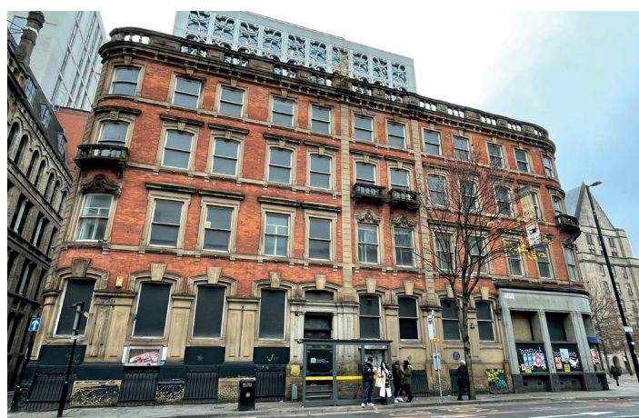
Image: Princess Street elevation, showing current situation with existing (altered) doorway to right hand side of stepped doorway, and window opening to left hand side of stepped doorway, currently boarded over.
