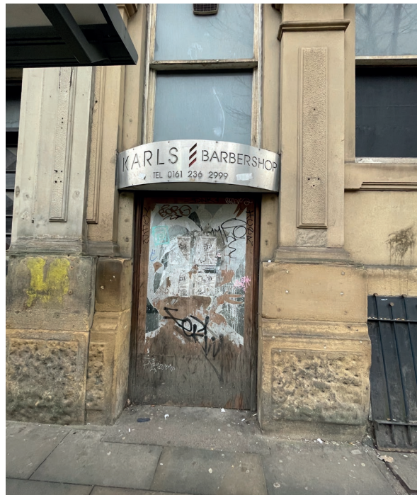
Image: Photograph of existing altered entrance to former barbershop unit, Princess Street.
