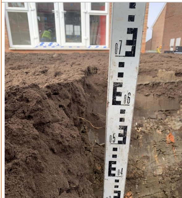
Depth of Cover System at Ground Level
