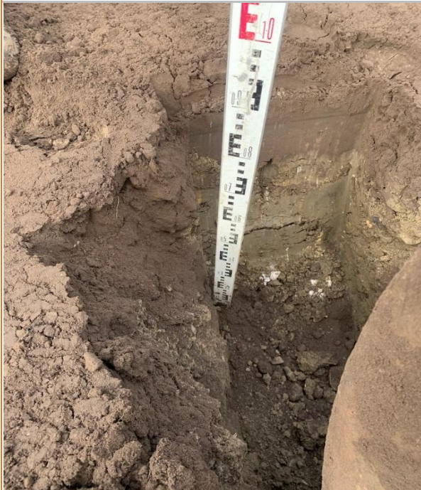
Depth of Cover System at Ground Level
