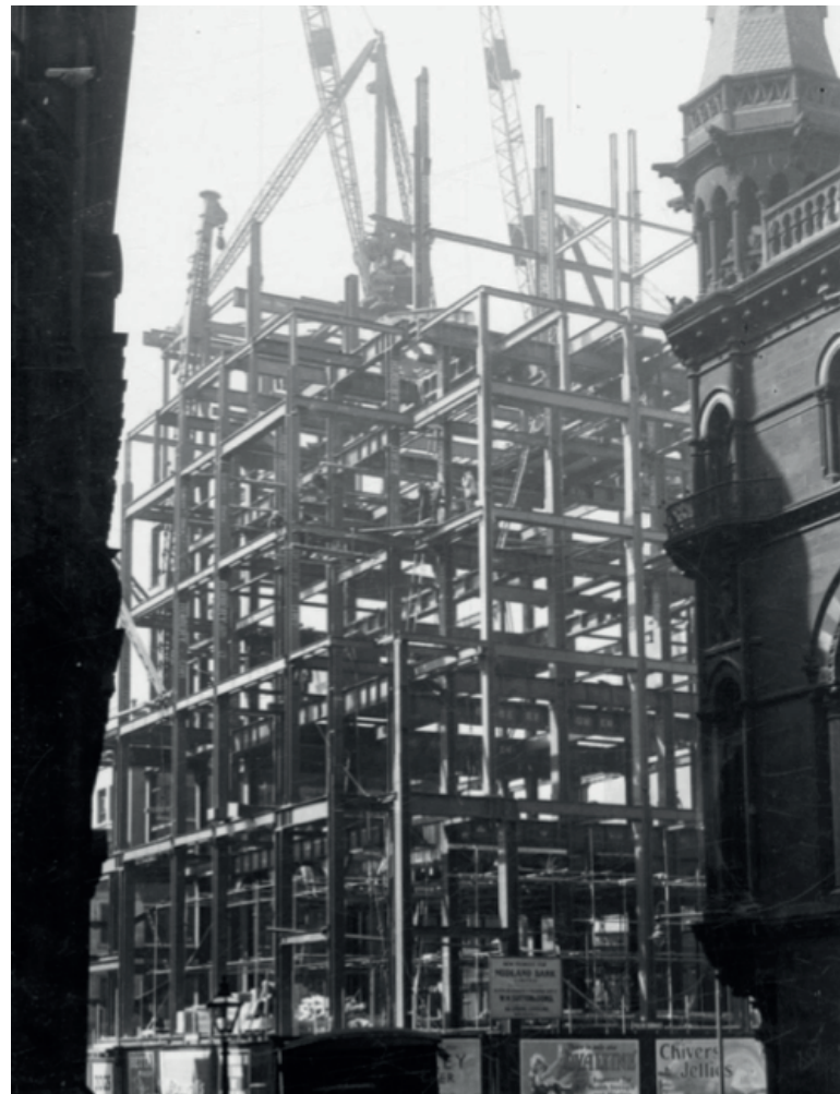
Image: The building during construction in 1929/30. (Manchester Archives).
