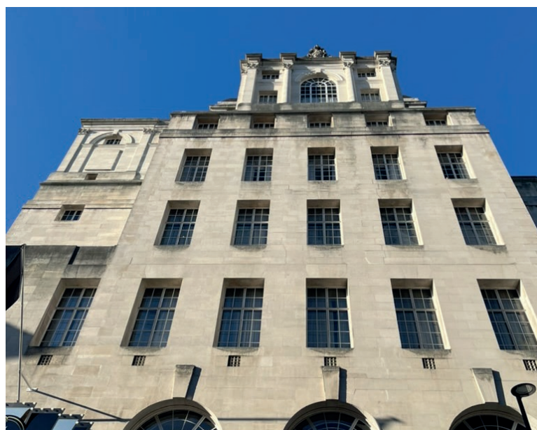
Image: External view of windows. Those at lower level have already been fitted with secondary glazing, which can not be identified from street level.
