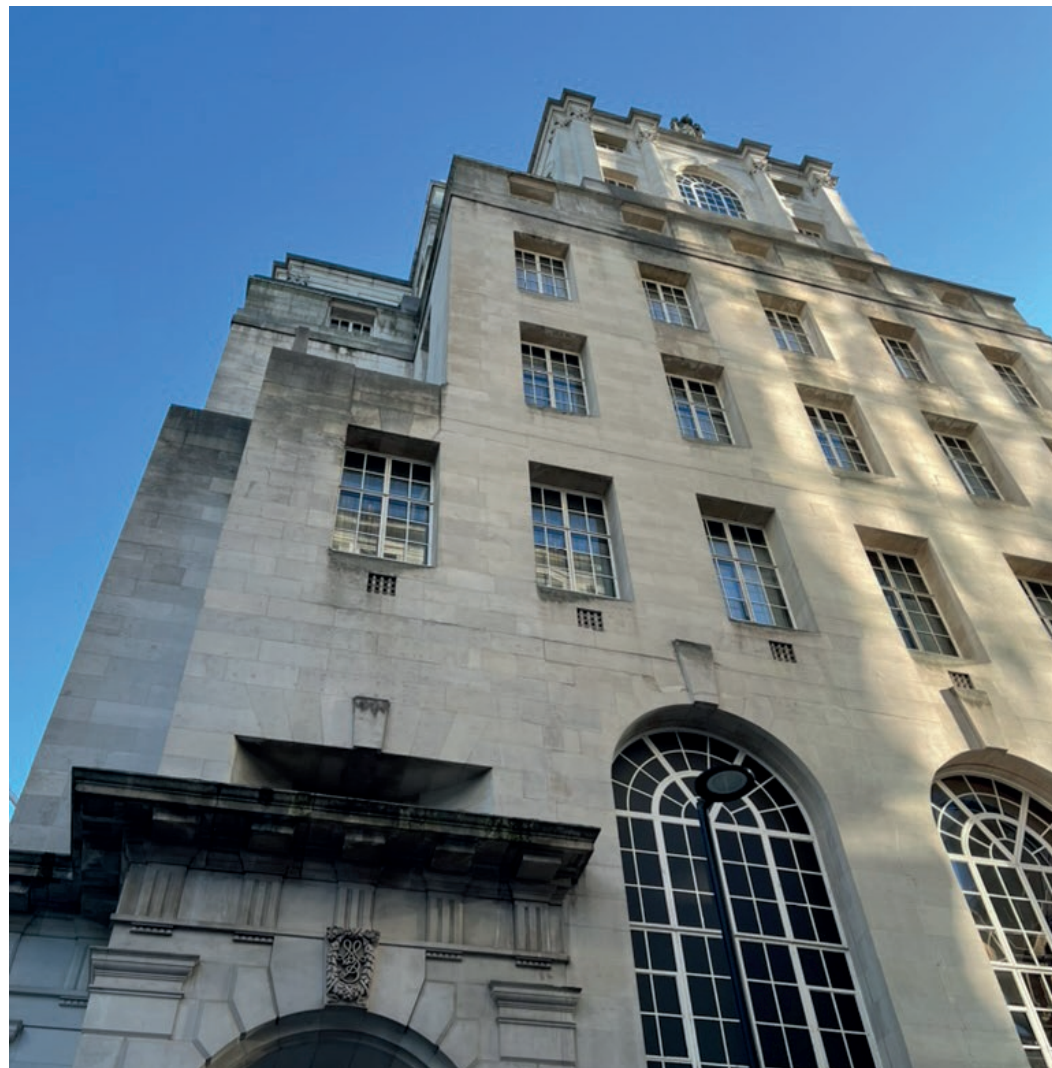
Image: 100 King Street elevation showing rhythmic placement of windows and deep reveals.
