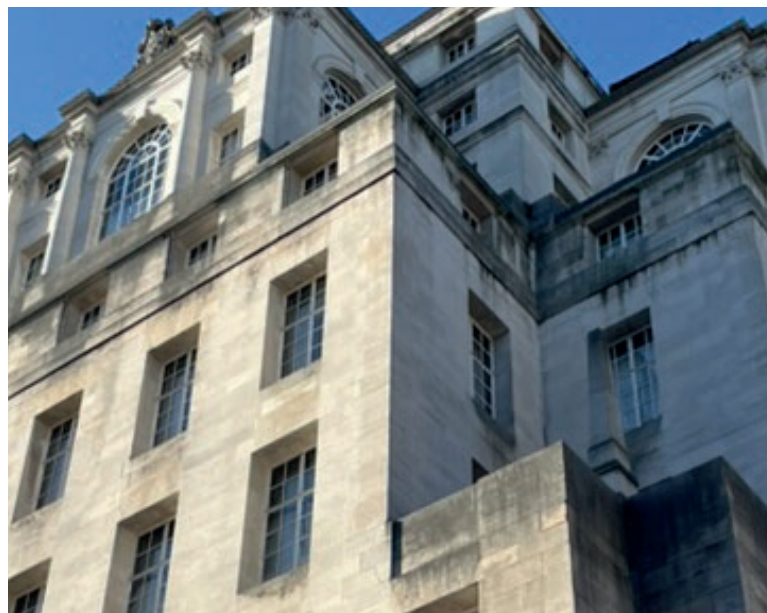
Image: External elevations of 100 King St. showing various sizes of windows. Those to the 4th floor can be identified by their more squared shape.
