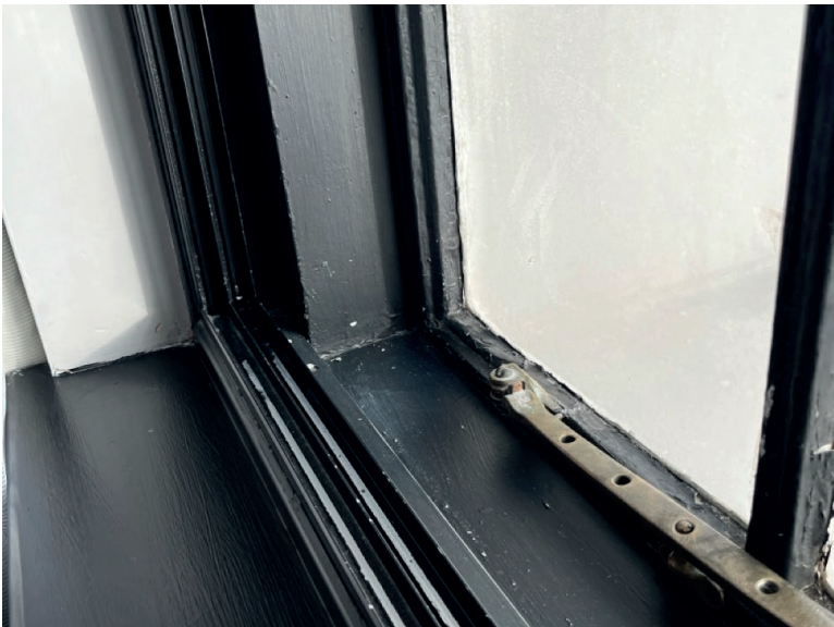
Image above: Example of window type. Image below: Example of existing secondary glazing, fitted in limited instances.
