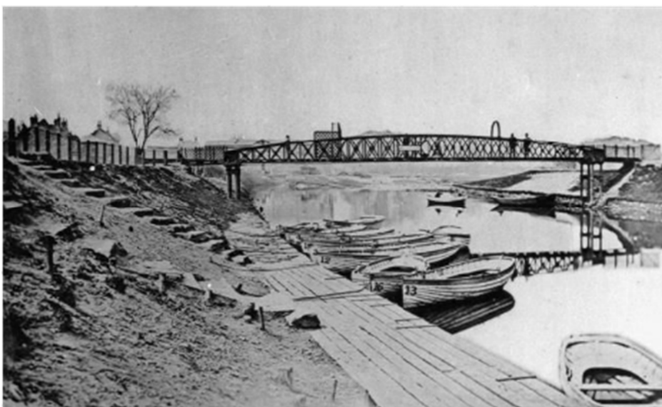
First iron footbridge bridge over the Mersey built around 1863.
