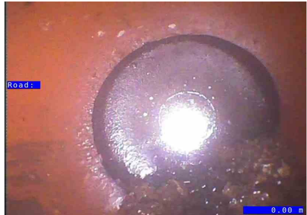
L2X_c8be1bea-a494-48c5-9e11-209e96547c49_20251203_1 03807_670.jpg, 00:00:16, 0.10 m Survey abandoned, Capped off
