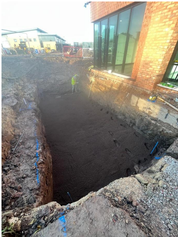
Figure 2 - Attenuation Tank Photographs
