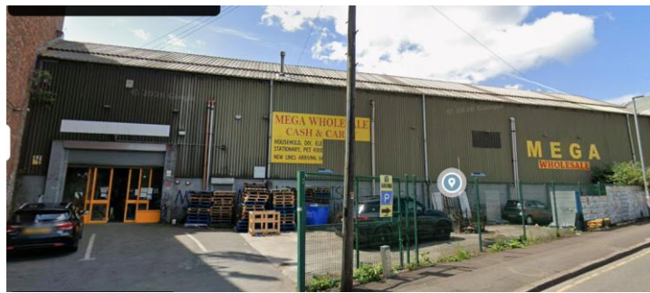
Existing Mary Street elevation to be overclad
