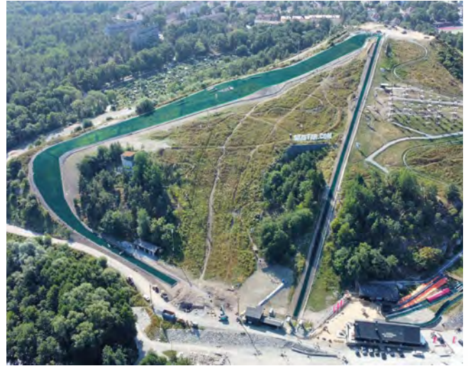
Moving Carpets, Dry Slopes, Summer Tubing, and Mountain Coaster in the middle of Stockholm (Sweden)
