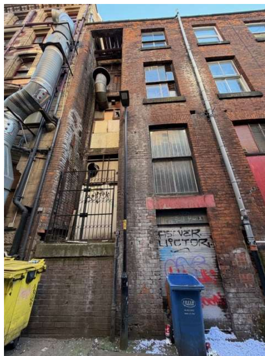
Figure 2 – Rear Elevation of Building
