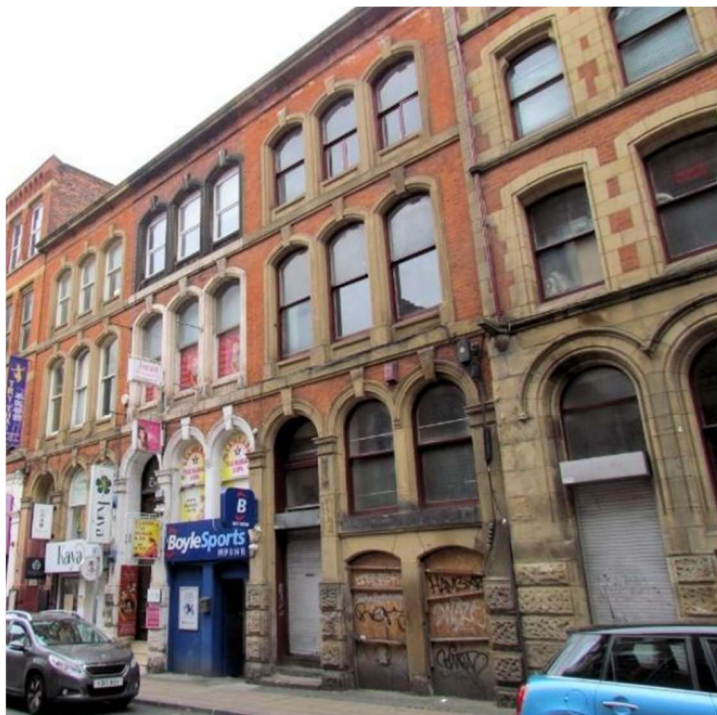
Figure 1 – Front Elevation of Building
