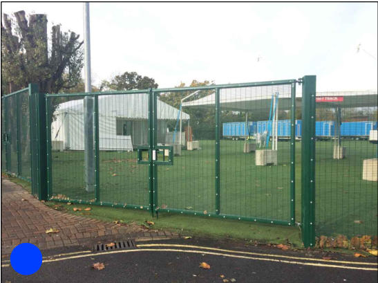
GATE Type 1 - Vehicle Access (#7) Double Leaf swing, style matched to fencing type location. Manual operation, fitted with drop bolts and lockable sliding latch
