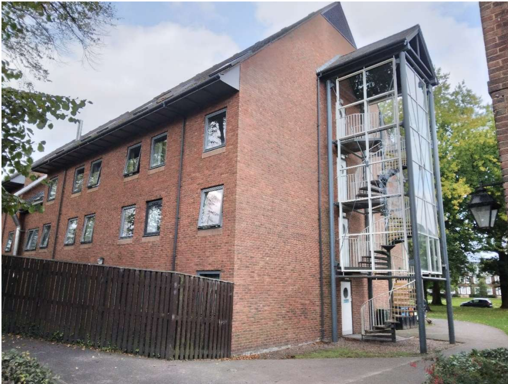
Photograph 3: Existing South Elevation
