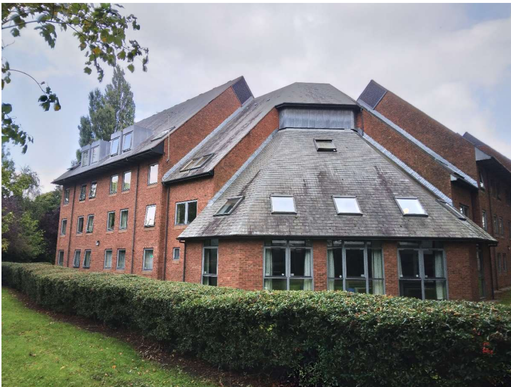
Photograph 6: Existing West Elevation
