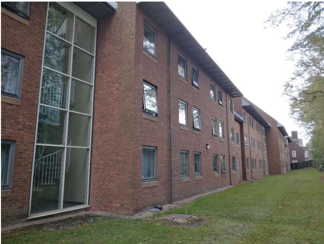
Photograph 4: Existing South Elevation
