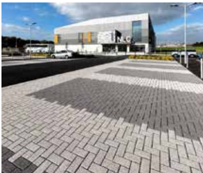
Permeable paving - parking
