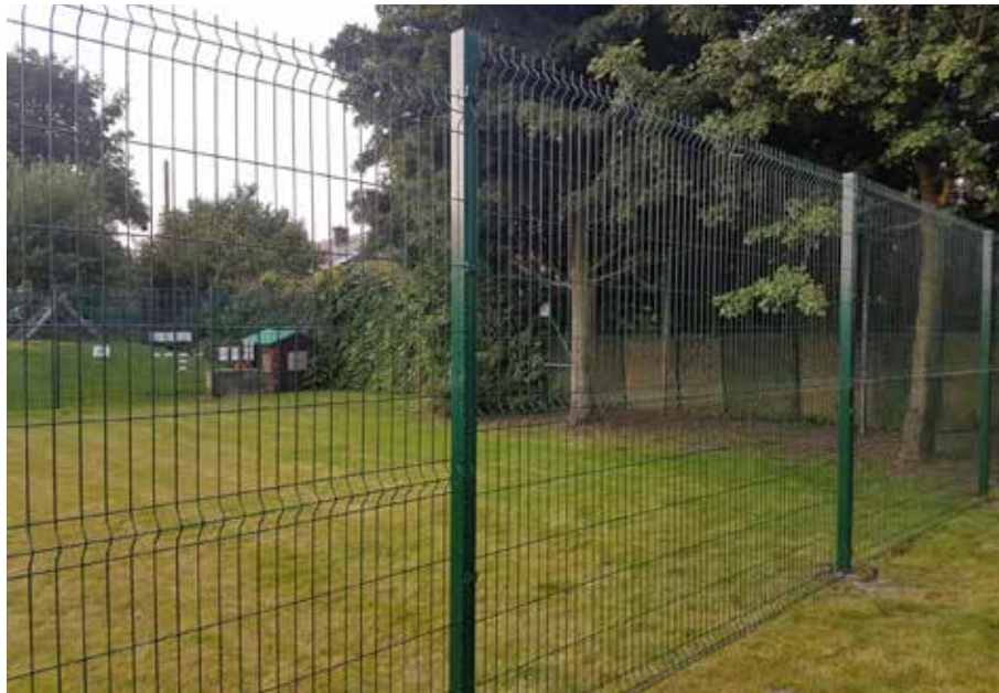
2.4m Weldmesh Security Fence
