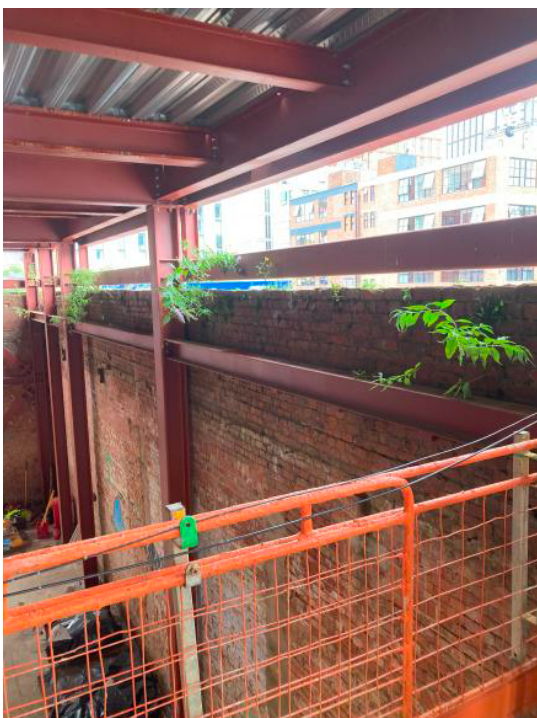
Removal of plant growth and treat
