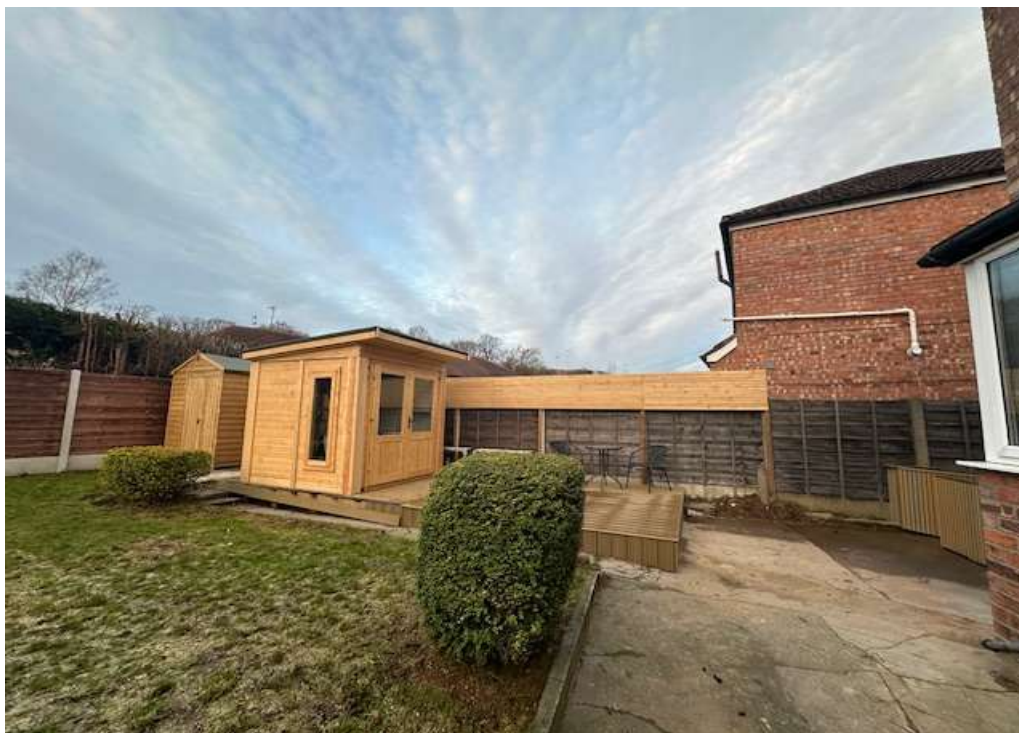
Figure 2: Photograph of retrospective development; raised platform, shed, outbuilding, additional boundary treatment to northern side boundary and within the site curtilage.
