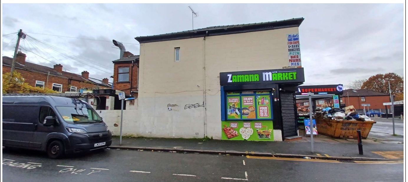
Application site in November 2025
