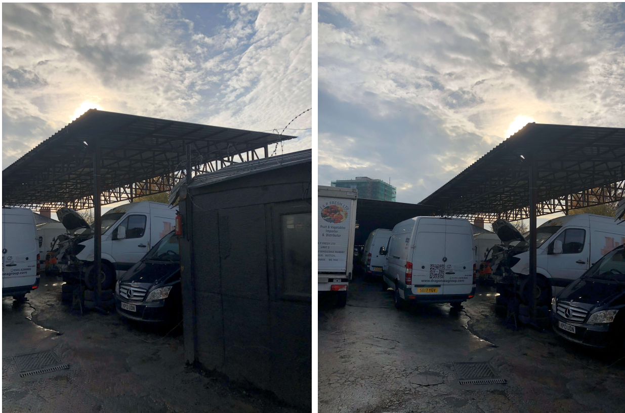
Figure 1, Canopy subject to the current application, as seen on site
