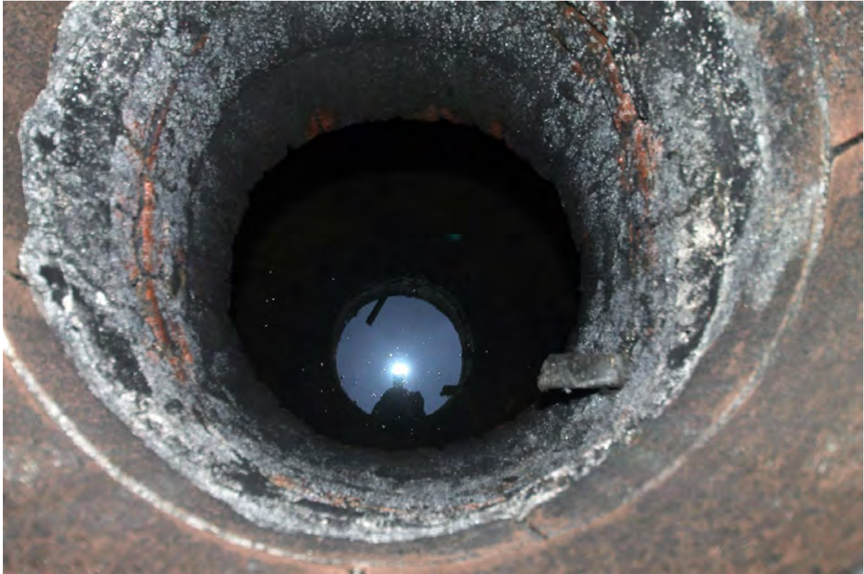
Plate 14. Wellhead, following removal of middle level, viewed from west. Note flattened lead pipe on right side of shaft, which probably connected to a pump.
