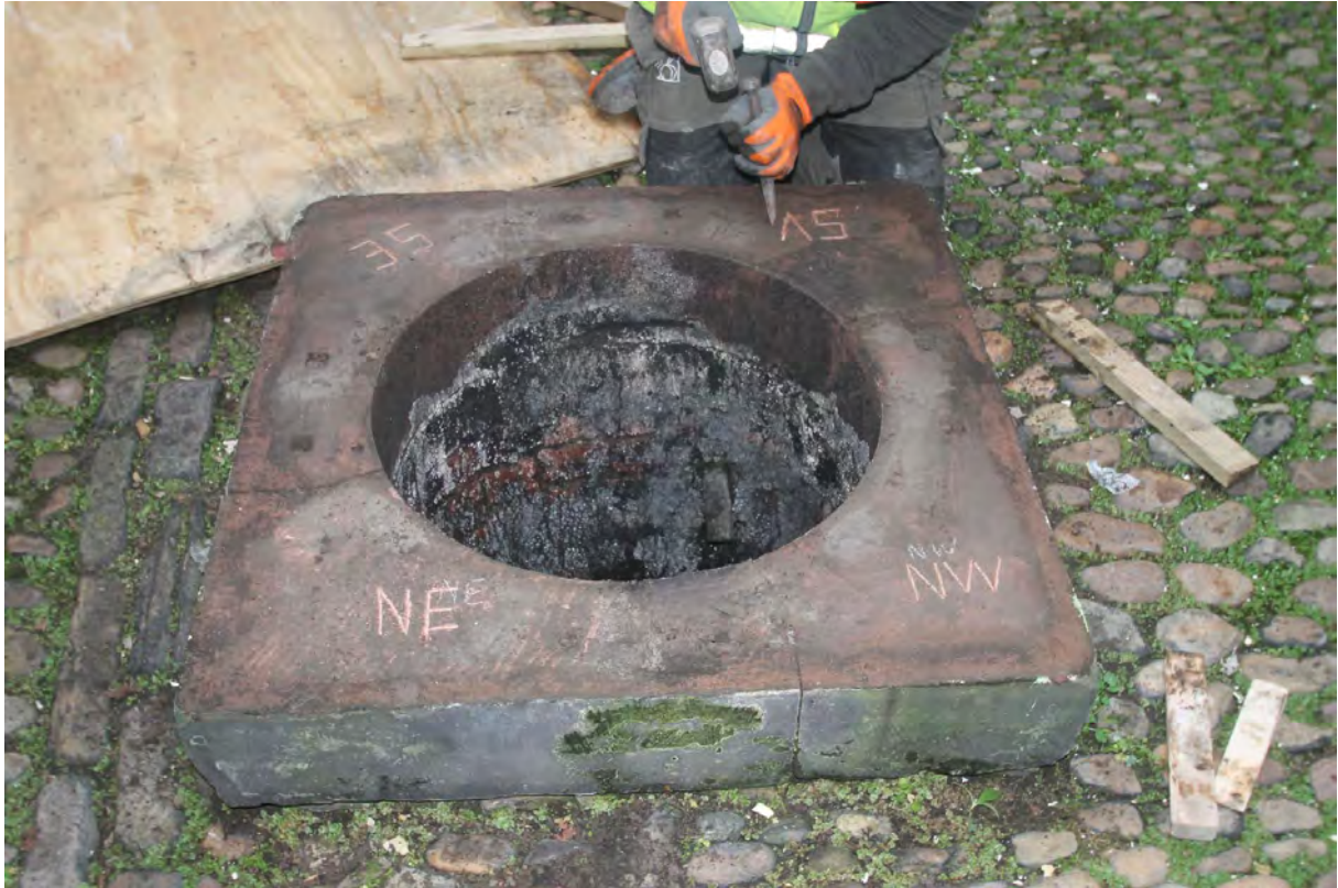
Plate 12. Wellhead, following removal of middle level, viewed from north.
