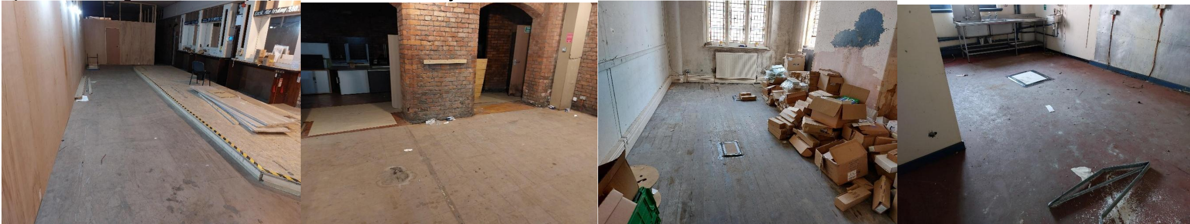
Flooring to be removed to access the void
