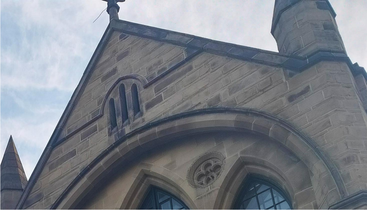
Figure 2-5 2025 from ground level. Shows joints have been mortared up to reinstate intended load paths & weather tightness.
