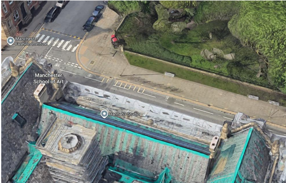
Figure 2-13 Satellite showing rear of gable elevations. Western gable (left in view) with arch separation. Eastern right (right in view) without evident separation but still 1:50 lean.
