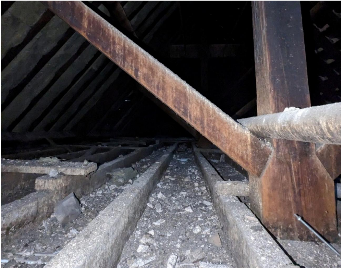
Figure 2-12 Inside Roof void space (Eastern gable) showing ceiling joists spanning between gable & King post trusses
