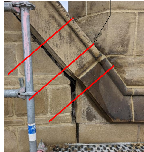
Detail 2- Local coping stone tying over crack SCALE: NTS
