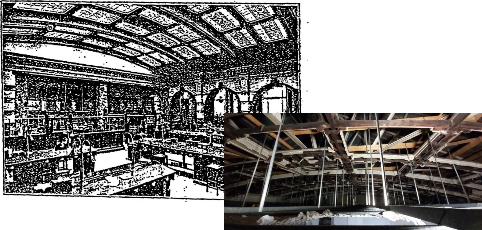
Fig 9: LEFT The only record photograph of the former clerk's hall, from The Builder's Journal 1907; RIGHT photograph taken looking across the current ceiling void showing only the timber primary ceiling structure still in place.
