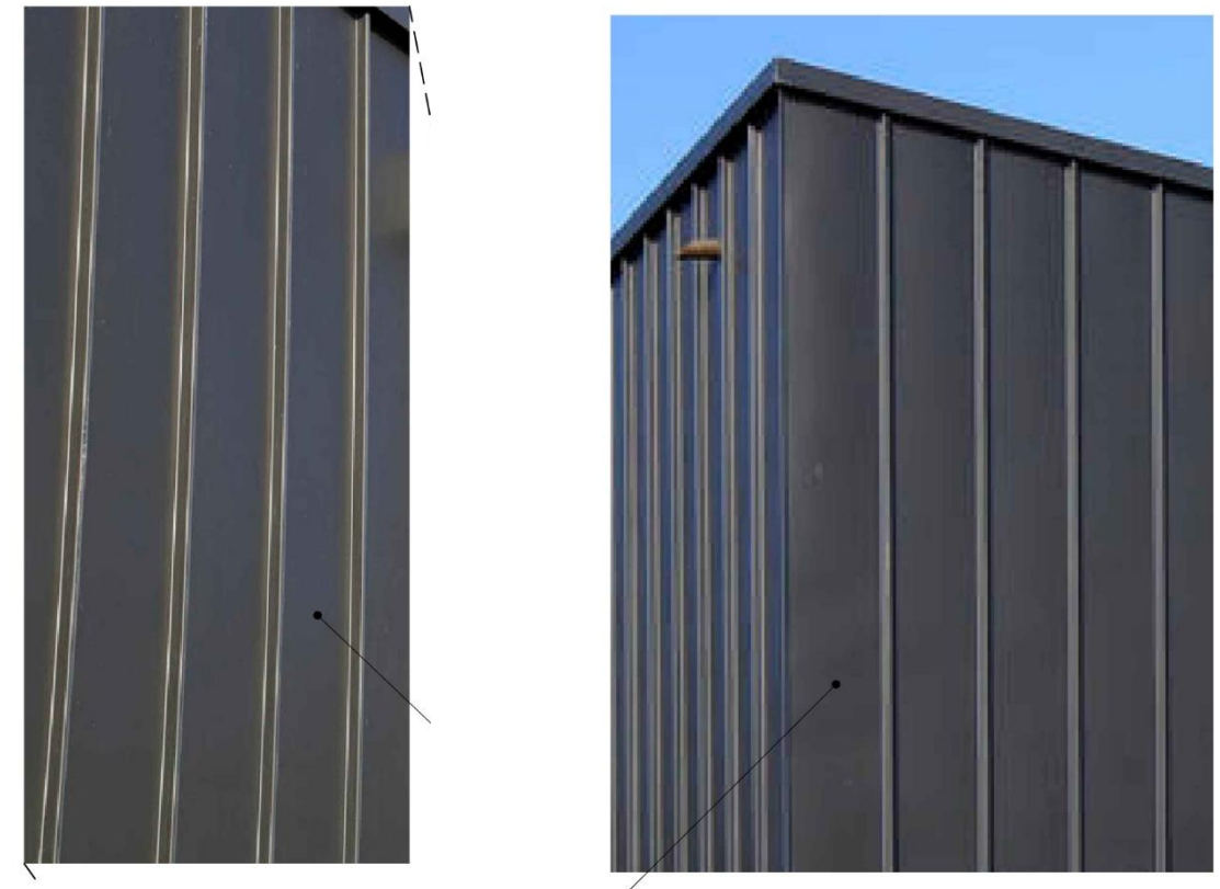
Fig 12: Images showing typical dark finish coated zinc cladding.
