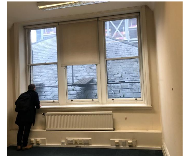
Fig 19: Typical window showing wide mullion sections between sash casements, and radiator & services boxings to be removed.
