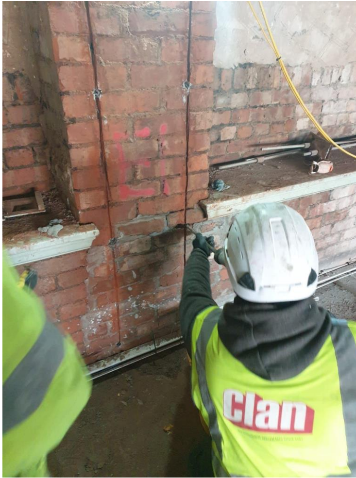
Photograph 3: Close-up view of chases and drill holes for anode mortar installation
