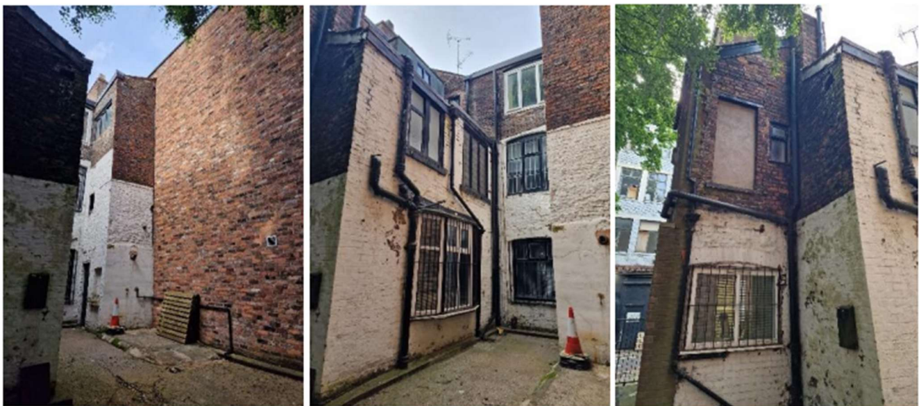
Figure 6 – Existing photographs of rear/side projections
