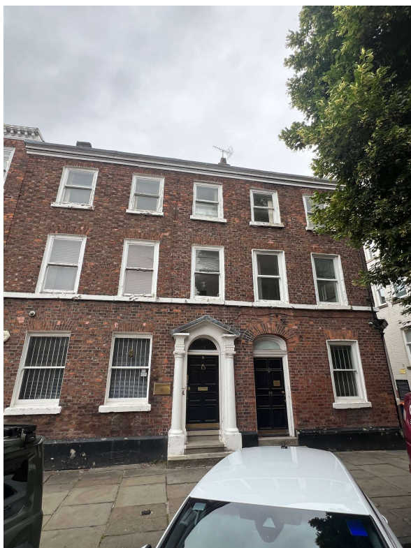
Figure 1 – Front elevation of listed building
