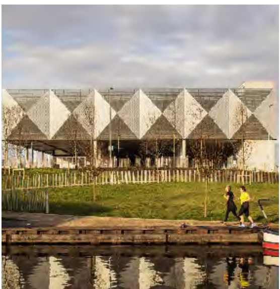
3D facade elements: Leeds University, CJCT Queen Elizabeth Park, London, Haptic
