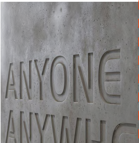
3. Precast Concrete Core with cast in signage
