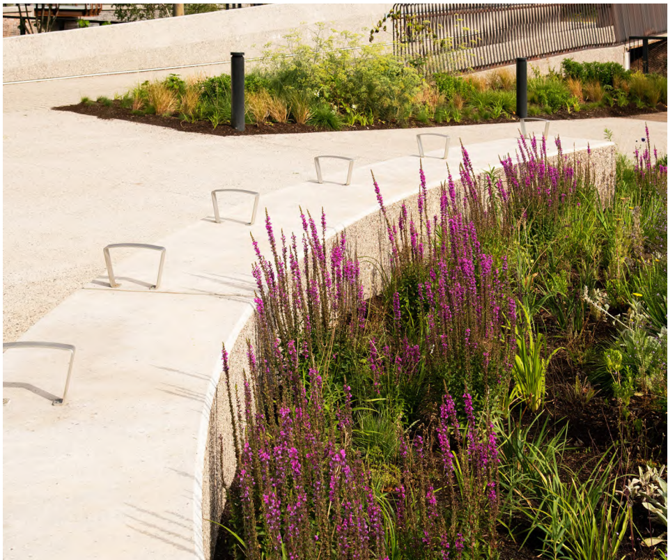
Rain Garden - Provides an opportunities to hold and soak surface water whilst increasing the variety of planting types
