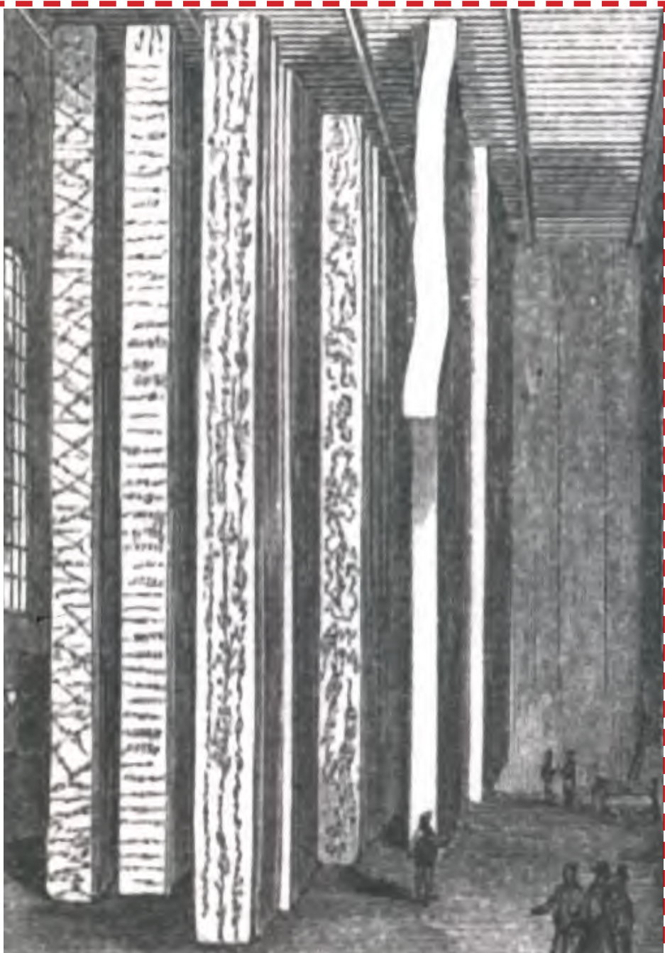
Historical image showing drying room at Hoyle Calico Printworks
