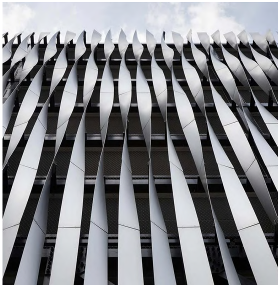
Hit and miss panelling: First Street, Manchester Car Park, Leeds, ACME
