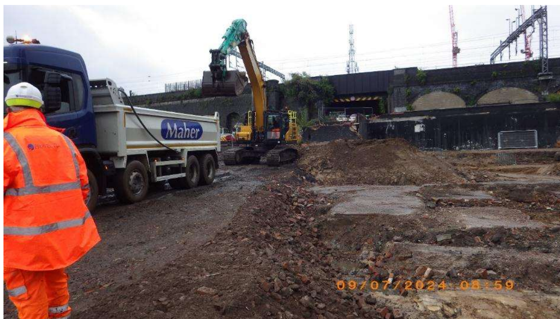
NT02: loading of TCE material (see Appendix J for further details)
