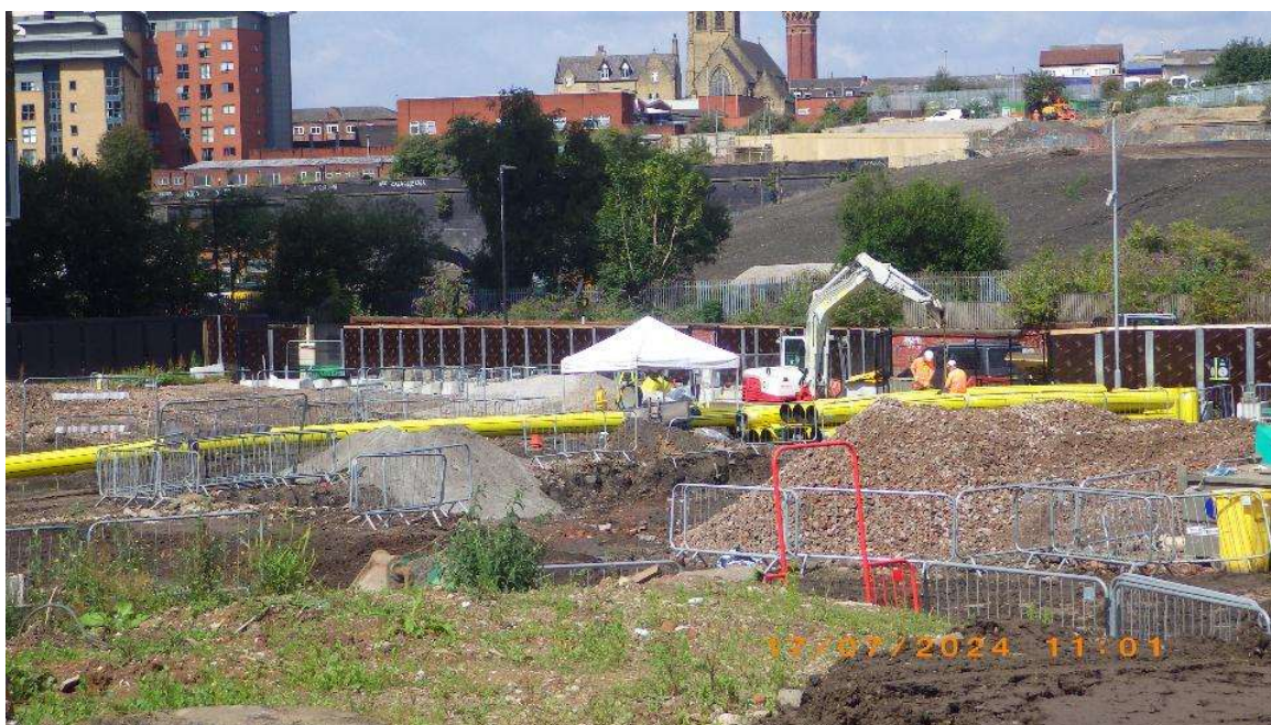
NT02: preparation for installation of MP gas diversion by Cadent
