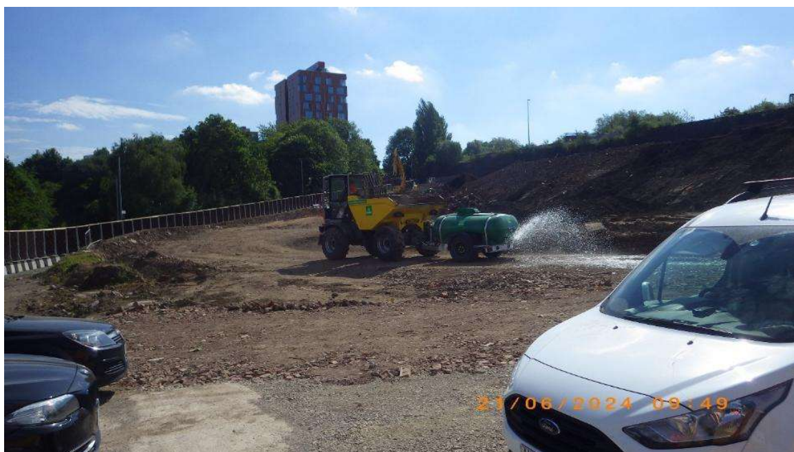
NT03/NT04: dampening down of haul roads
