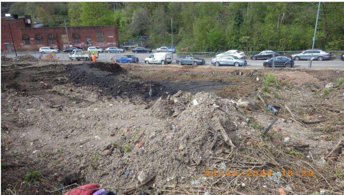
NT04, facing N towards Dalton St/Dantzic St junction
