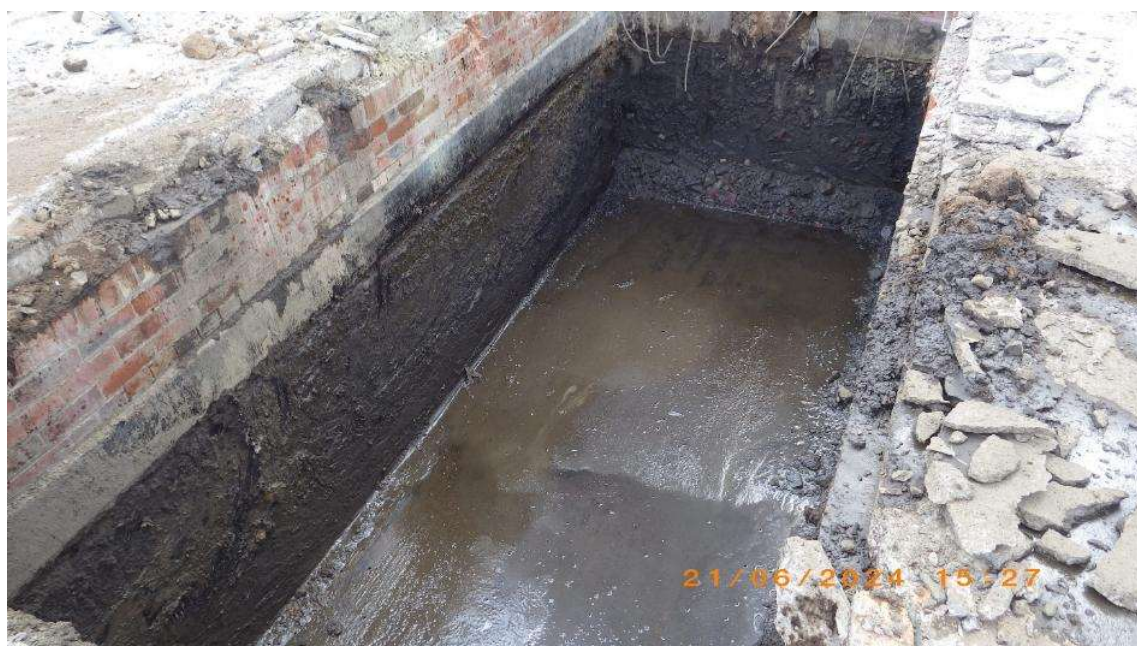
“NT02 tank” post-removal of water and solid contents
