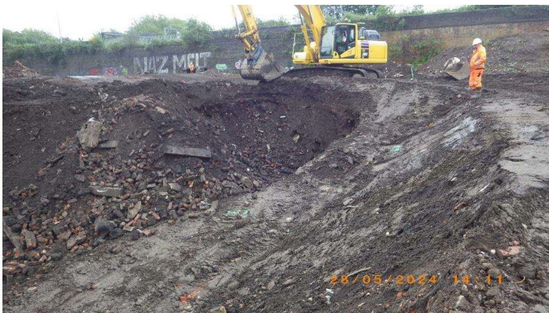
NT04 facing S: excavation works
