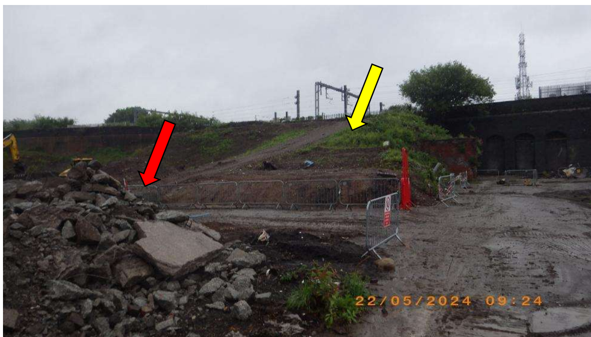
NT03 facing S towards railway viaduct. Note “ramp” (yellow arrow) and stockpiled oversize (red arrow)
