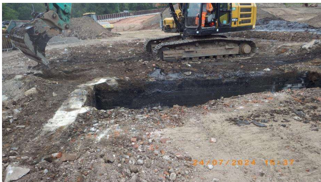
NT03: excavation and demolition of the wheelwash (see Section 4.1)
