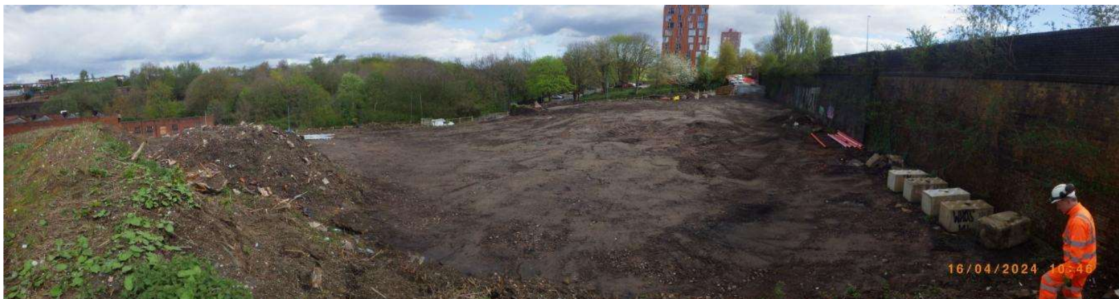
NT04: post-removal of majority of knotweed impacted material from E end towards Dalton St
