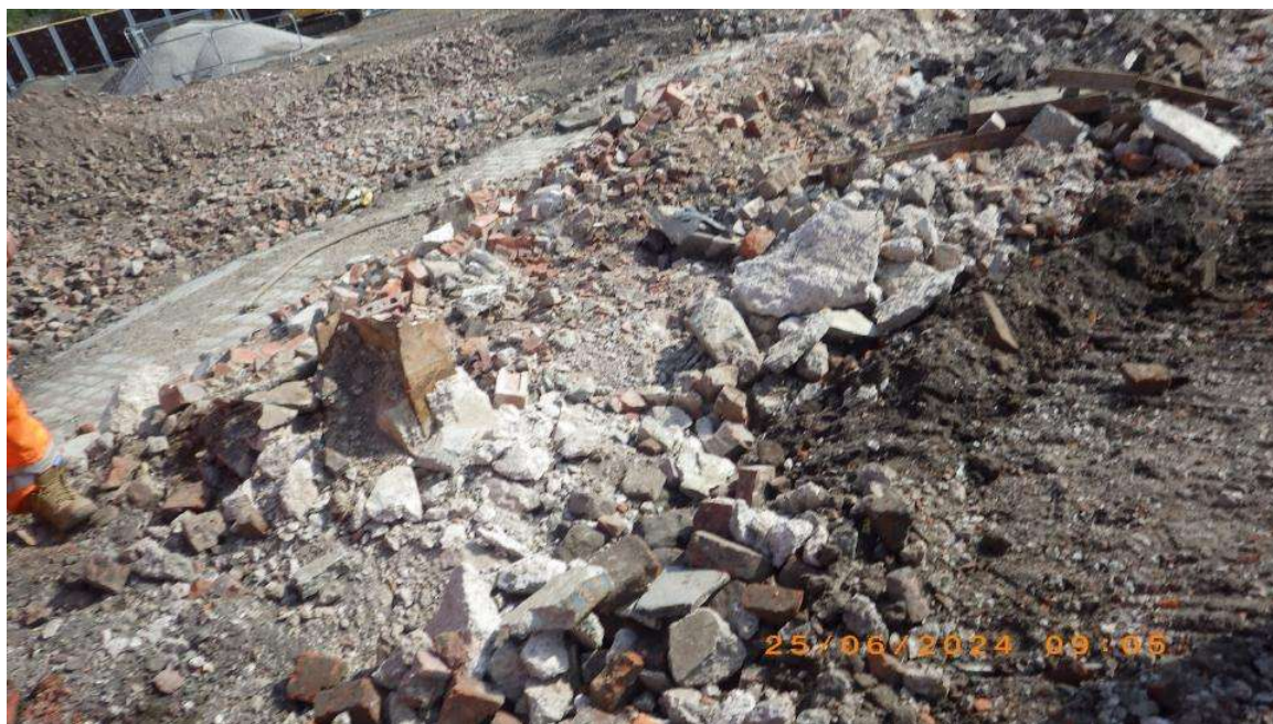
NT02: uncovering of obstructions (see Section 5)
