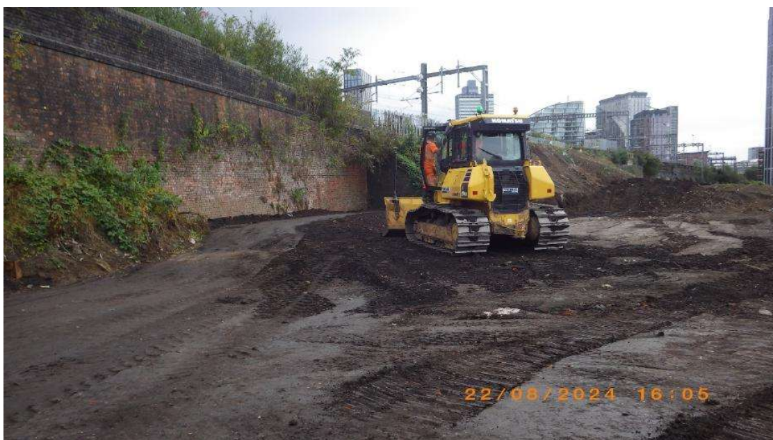
Placement and levelling of material between NT04 and NT03 to allow access to piling platform 22 nd August 2024
