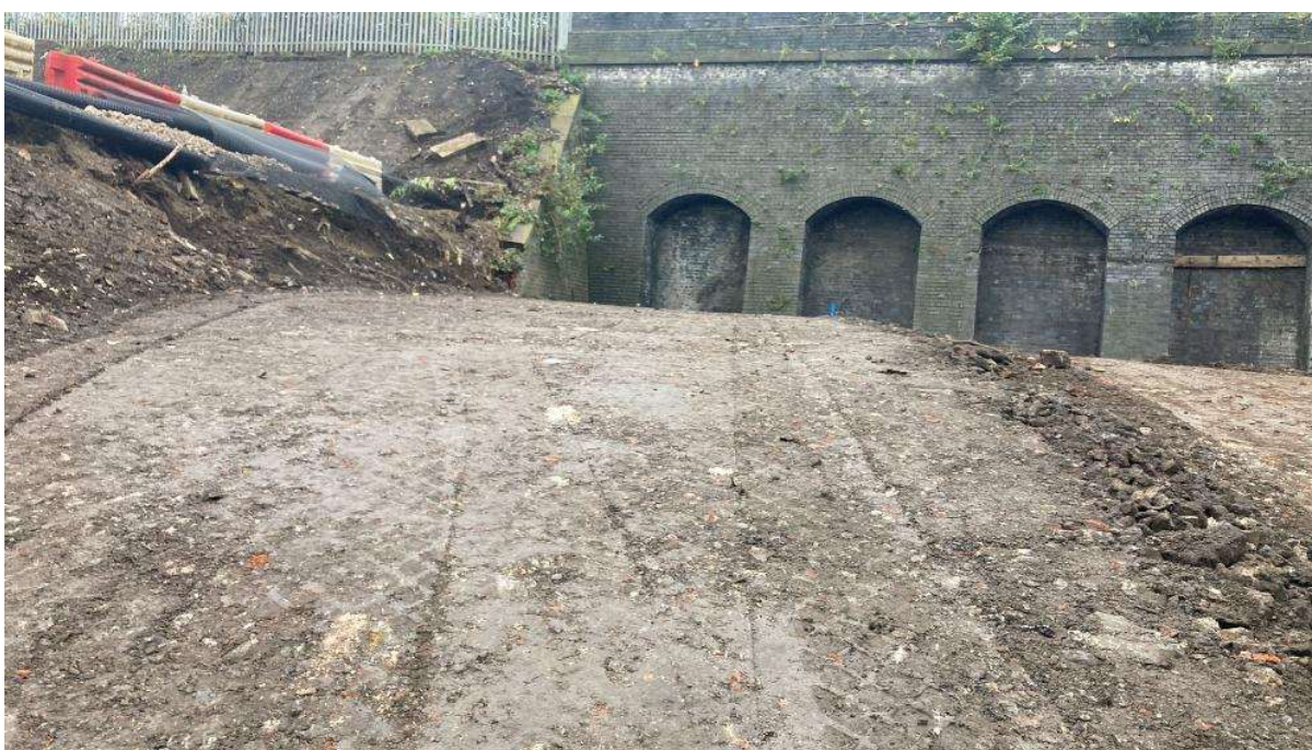
NT03 S boundary: extension of pile mat across area formerly occupied by MP gas main
