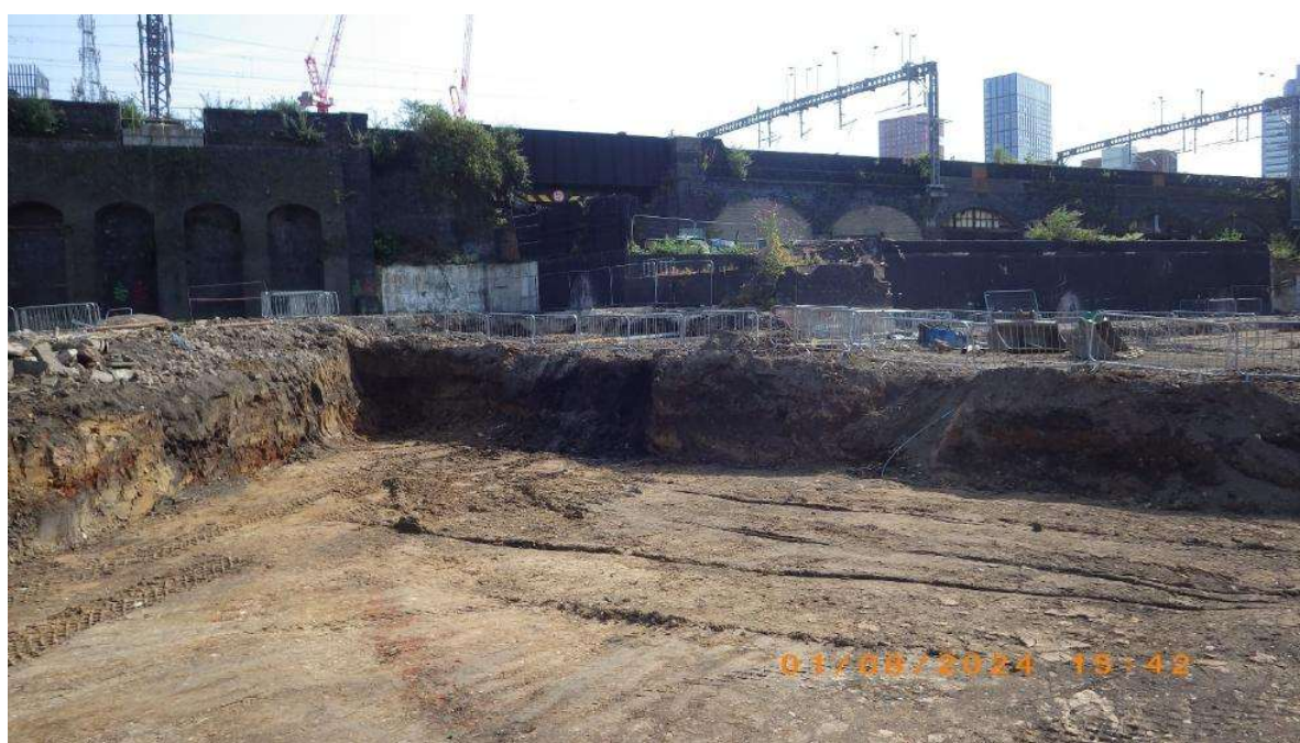
NT03: cutting of ash fill material. Material transferred to NT03 upfill area
