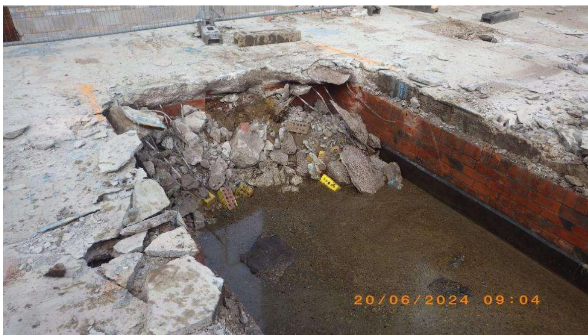
NT02 western boundary: "NT02 tank" encountered during demolition of floor slab
