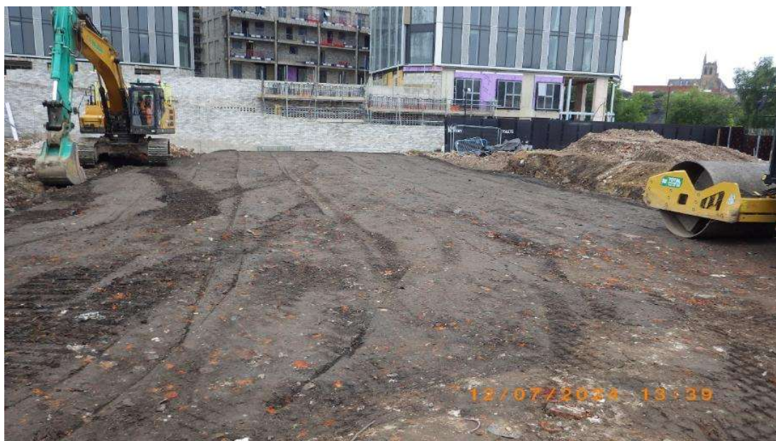
NT03: backfill and compaction following obstruction removal
