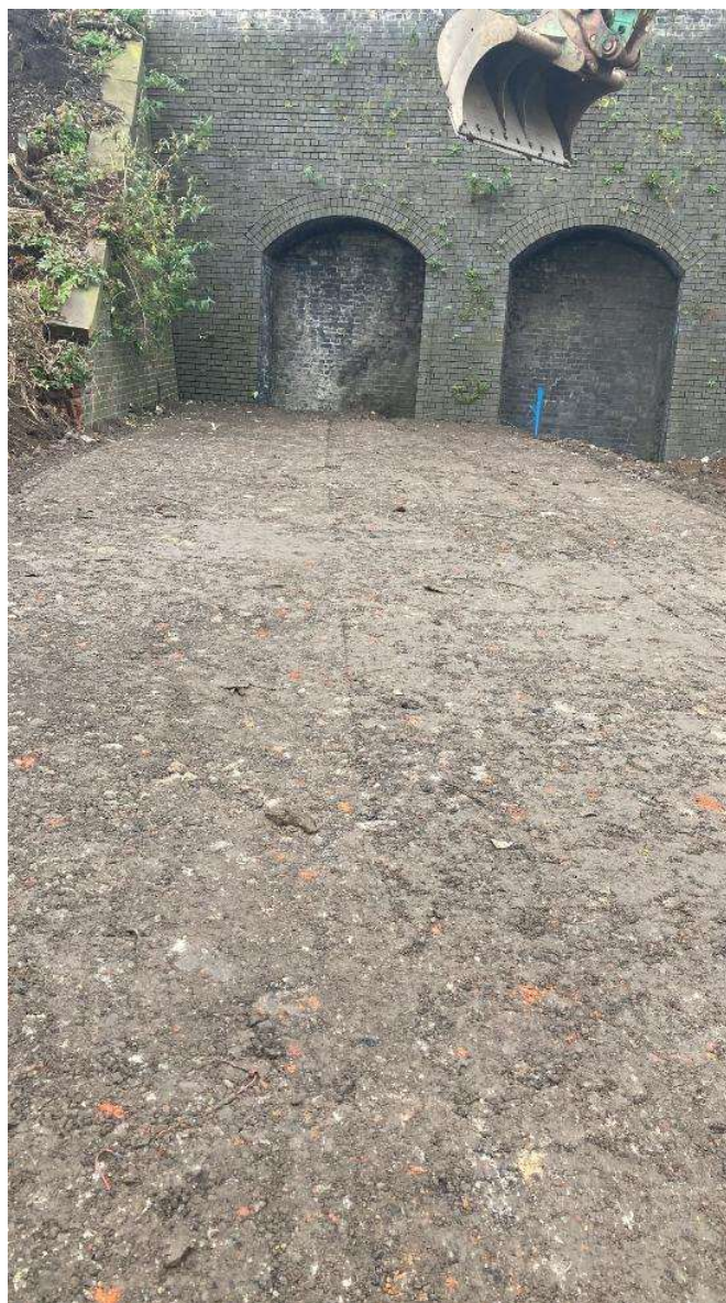
NT03 S boundary: extension of pile mat across area formerly occupied by MP gas main
