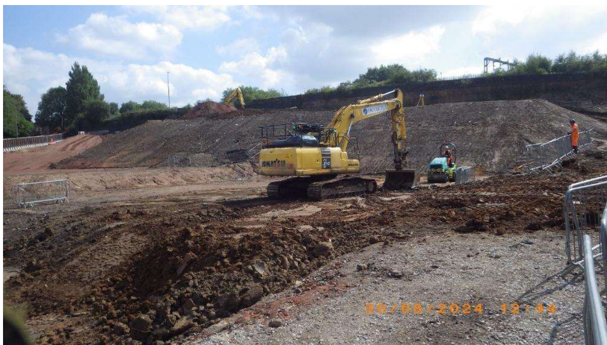
NT04/NT03, facing S: backfilling following chasing and excavation of redundant drainage
