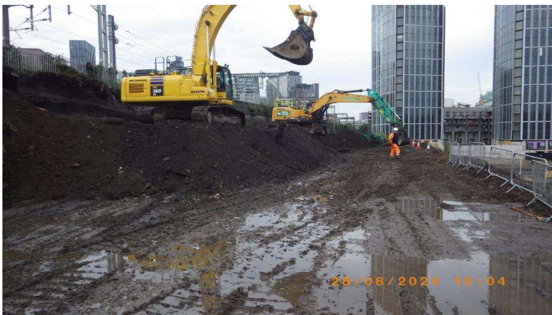
NT03, top of “ramp” on S border
