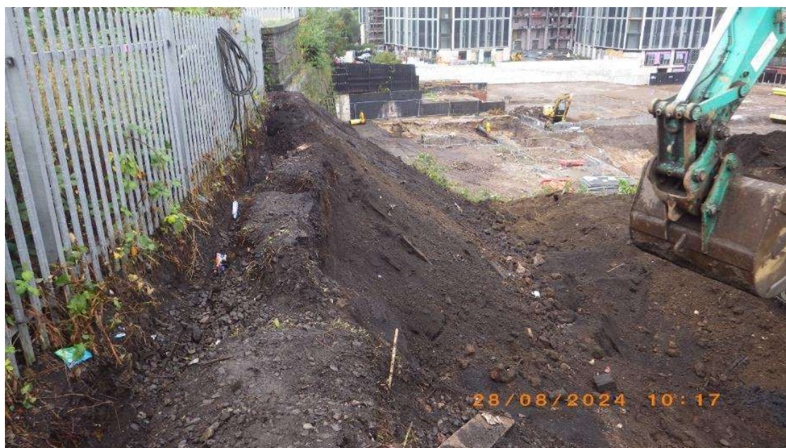
NT03, top of “ramp” on S boundary. Final cut.
