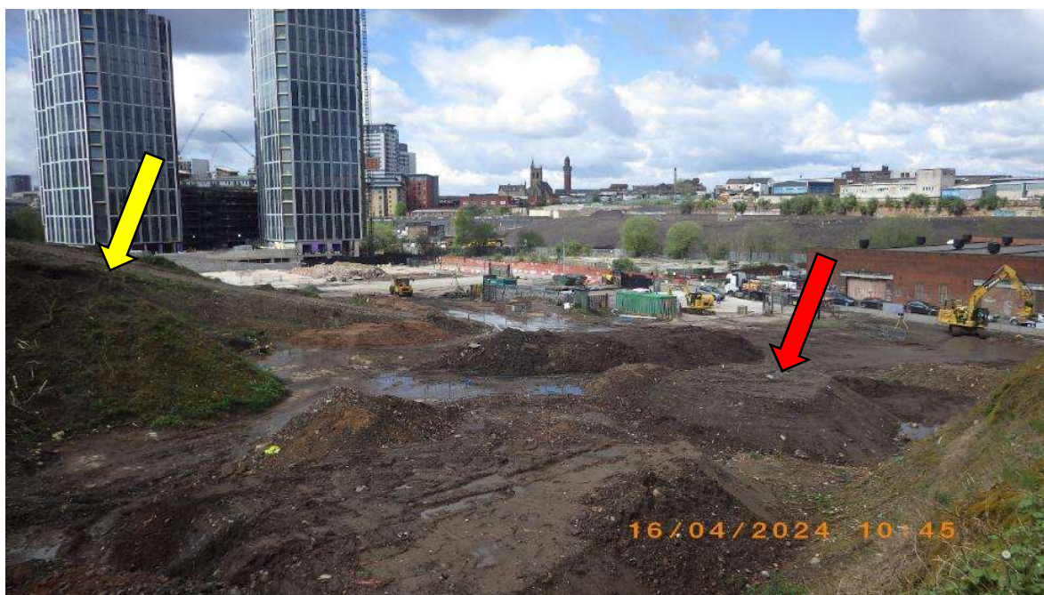
NT03 facing NW, prior to start of excavation works. Note “ramp” up to railway viaduct on site’s S boundary (yellow arrow) and “small piles” (red arrow)
