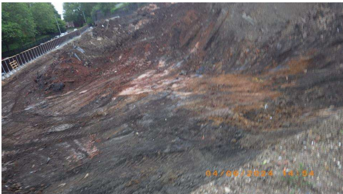
NT04 facing E. excavation & export cont'
