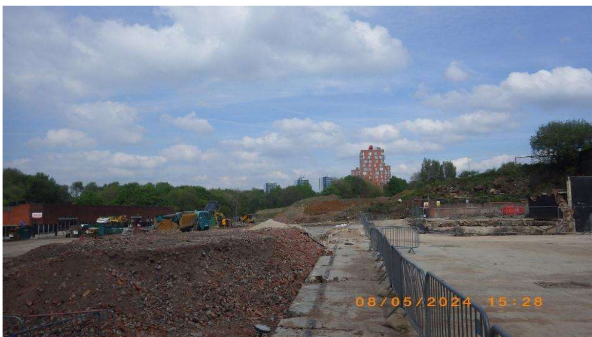
NT02 facing east...TCE area to right, 6F2 originating from original buildings' demolition stockpiled to left
