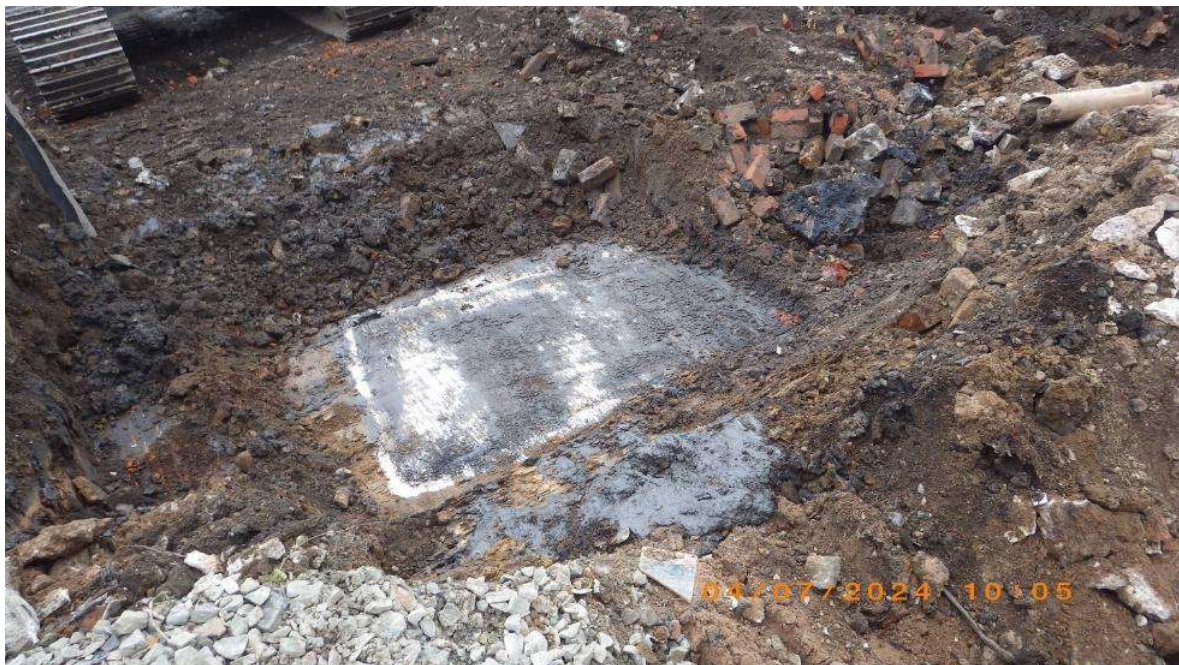
NT03 "small tank" demolition
