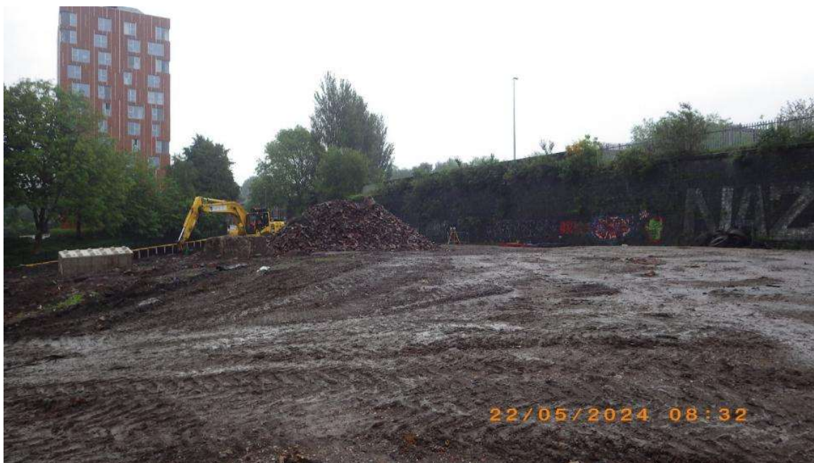
Facing E, demolition of redundant structure in NT04
