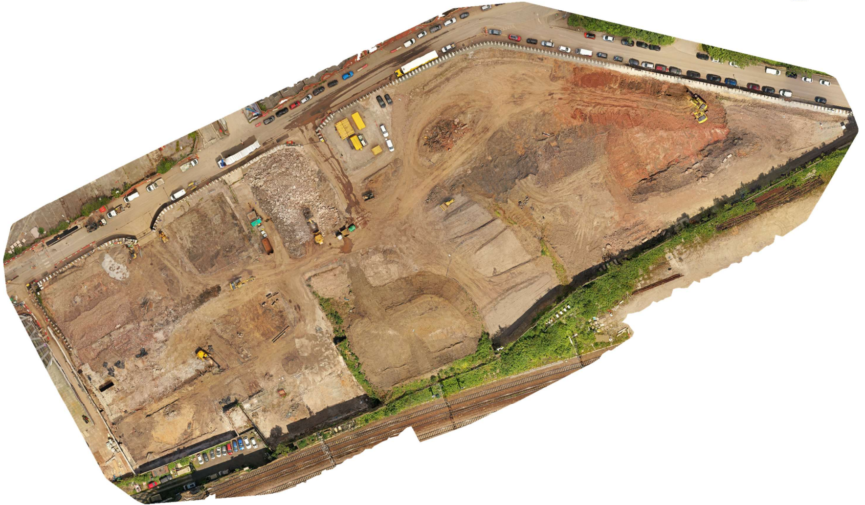
Site-wide drone photograph: 27 th June 2024
