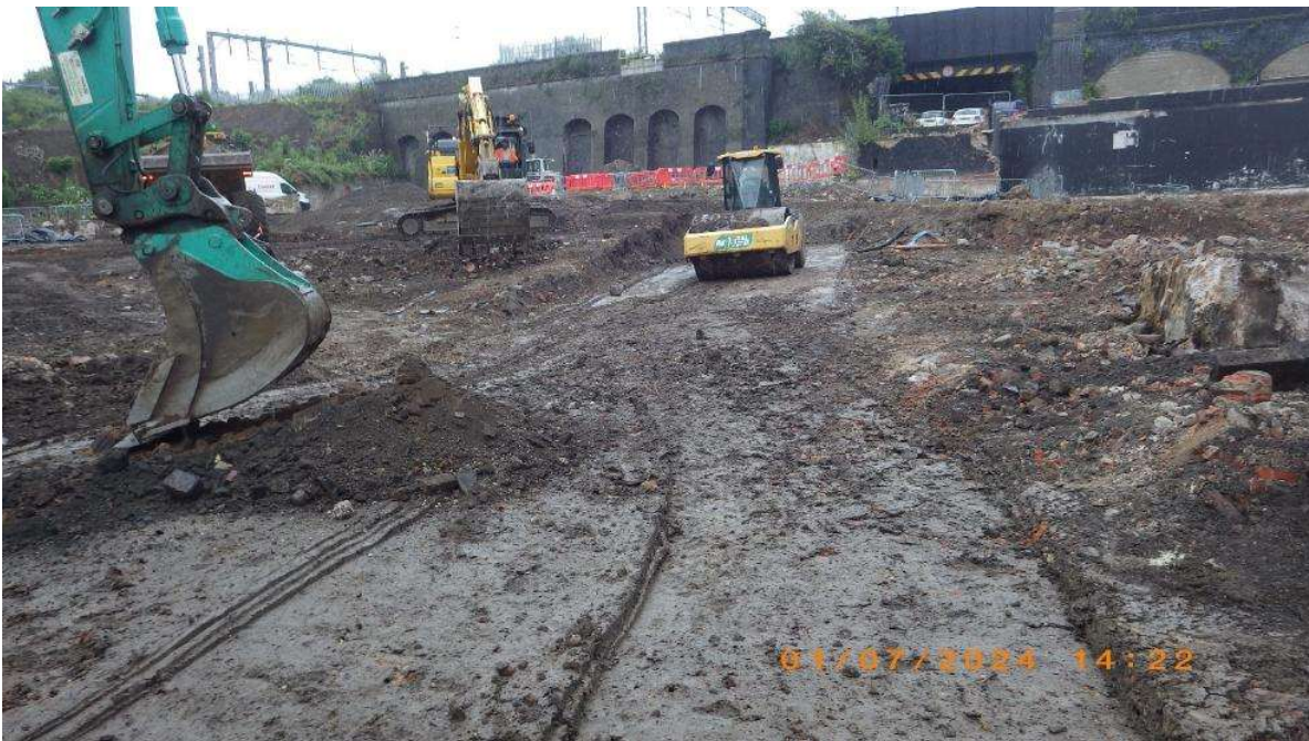
NT02: backfilling post drainage run chasing
