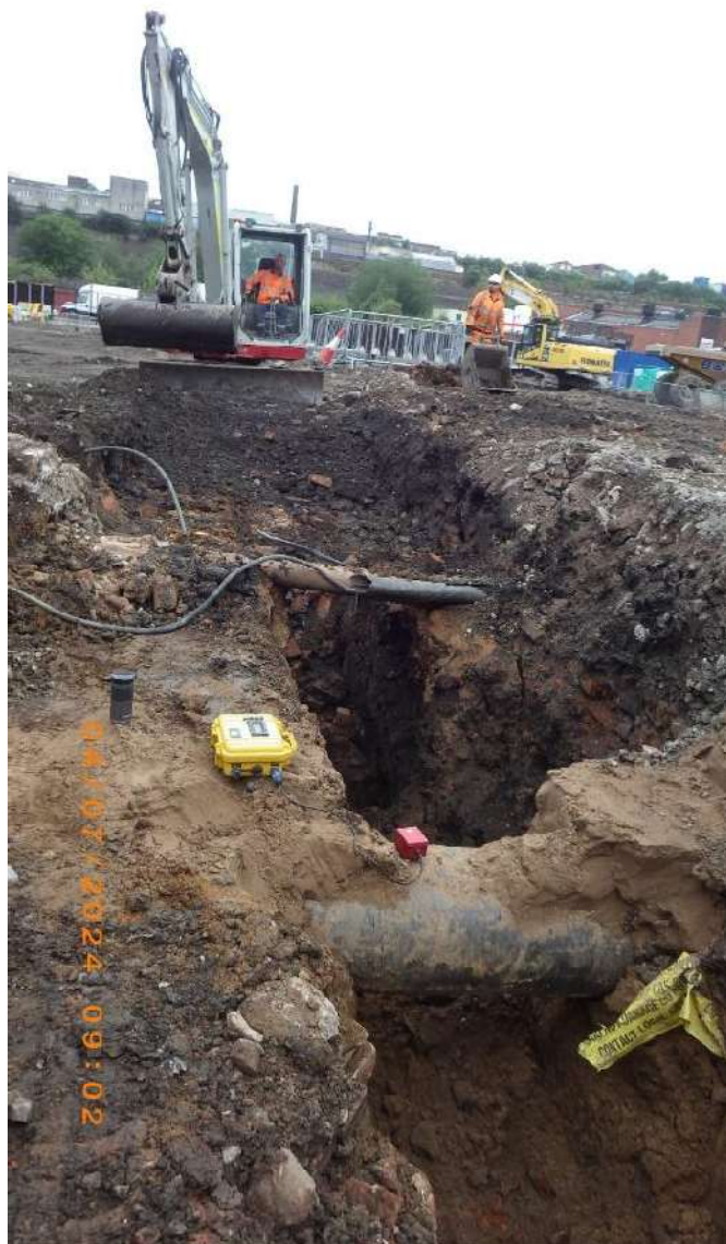
NT02: exposure of MP gas main by Cadent
