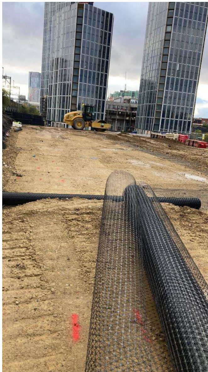
NT03: pile mat continues
