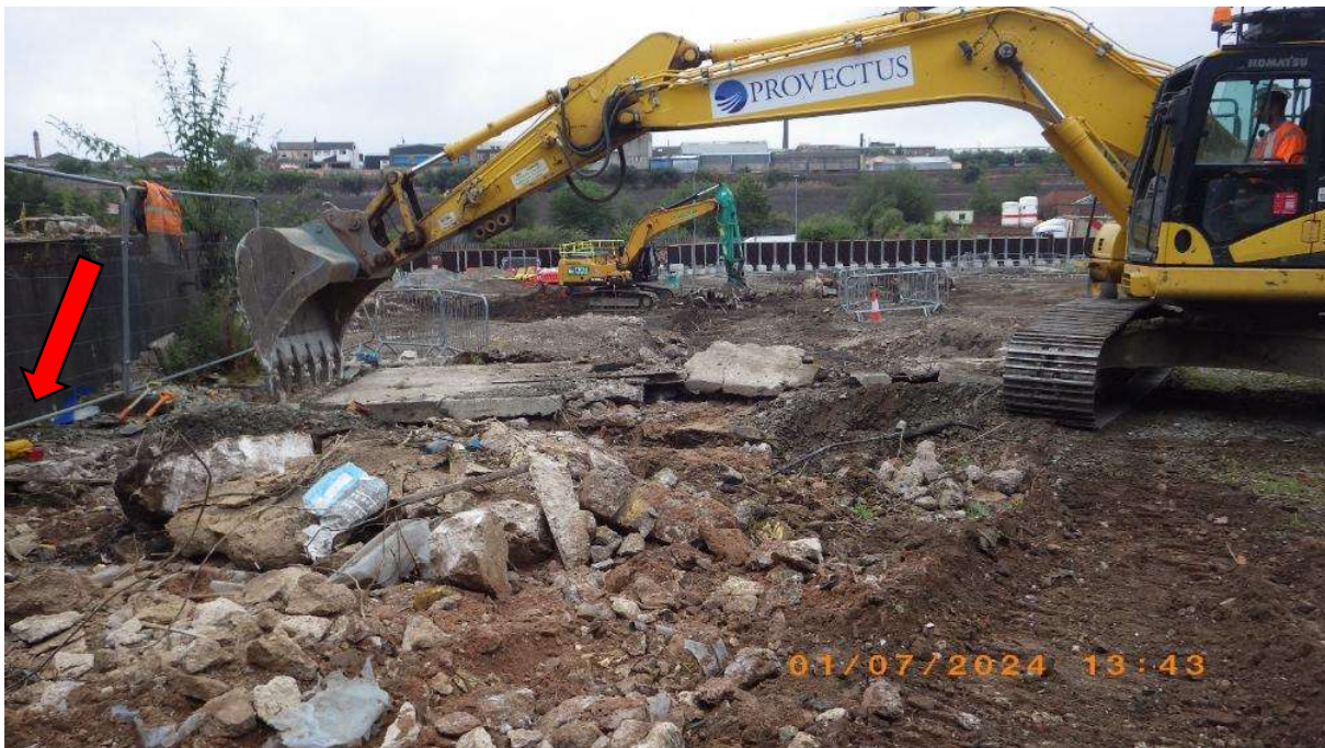
NT03: removal of the floor slab around the “small tank” and MP gas main (note vibration meter, red arrow on top of pipe)
