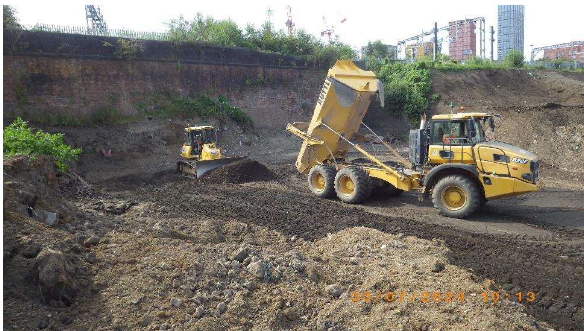
NT03: placement of material in permanent upfill area
