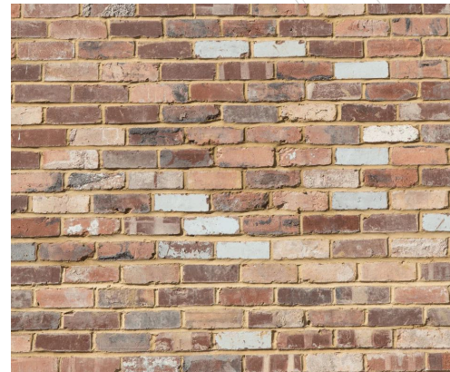
Image 1 - Precedent The image above illustrates the desired aesthetic finish for the existing boundary treatments.
