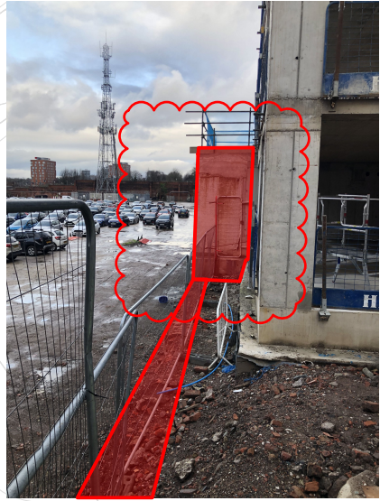
Wall A - Existing condition Demolished required rebuilding.
