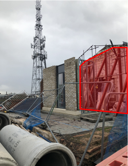
Boundary H - Existing condition Third party wall currently supported by piers.
