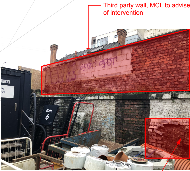
Wall D - Existing condition
