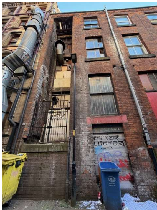
Figure 2 – Rear Elevation of Building
