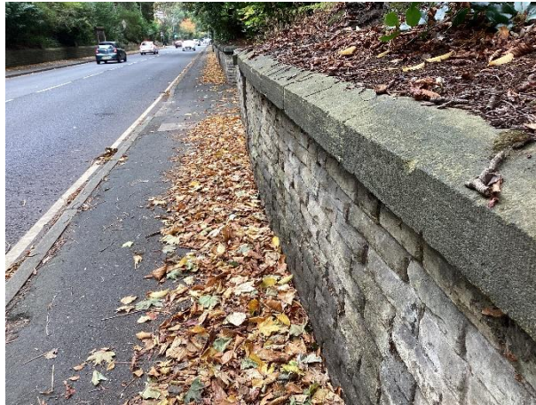
Note retained ground levels
