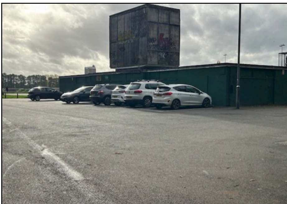
View of existing car park and building proposed to be demolished
