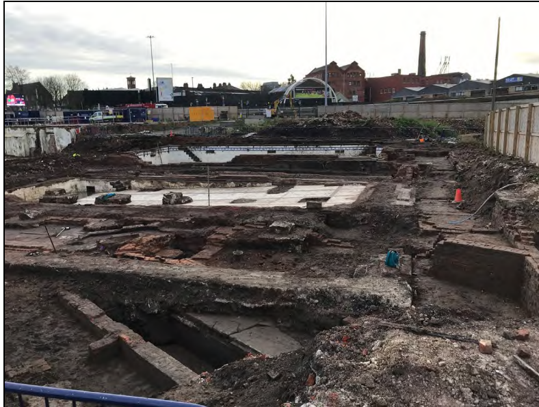
Plate 2.0: Mayfield Baths site following excavation
