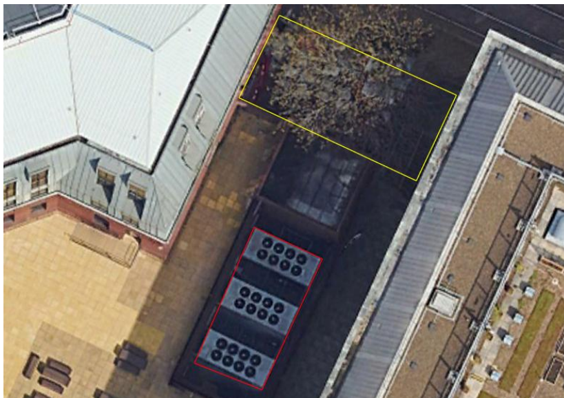
Figure 5 Proposed chiller compound location (yellow) and existing chillers (red)
