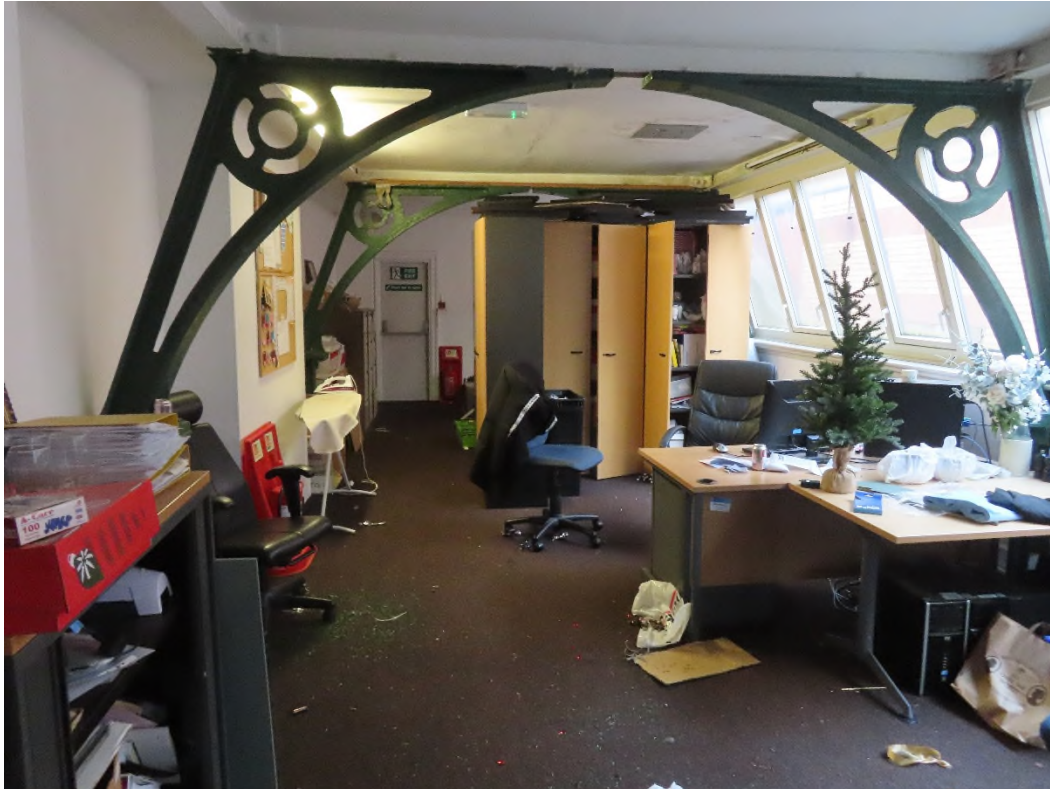
Indications of part of the steel frame exposed supporting the flat roof subdividing the front and rear building on the third floor.
