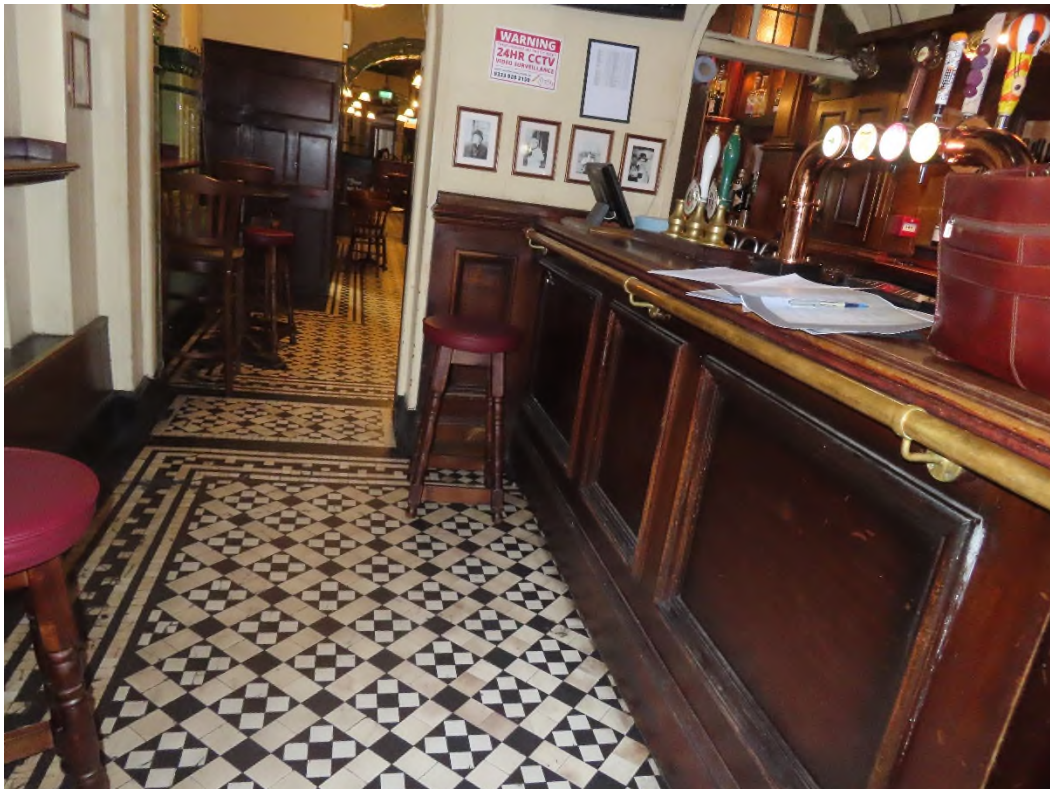
Existing bar to remain together with general refurbishment.
