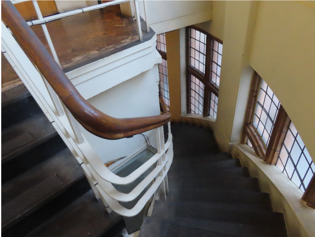
Detailed 1930's style balustrade to staircase remaining unaltered.
