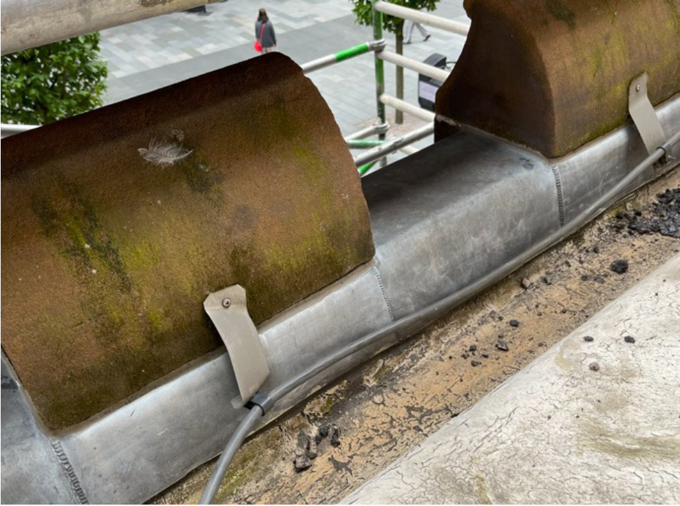
3.4 Asphalt Gutter with Lapped Lead
