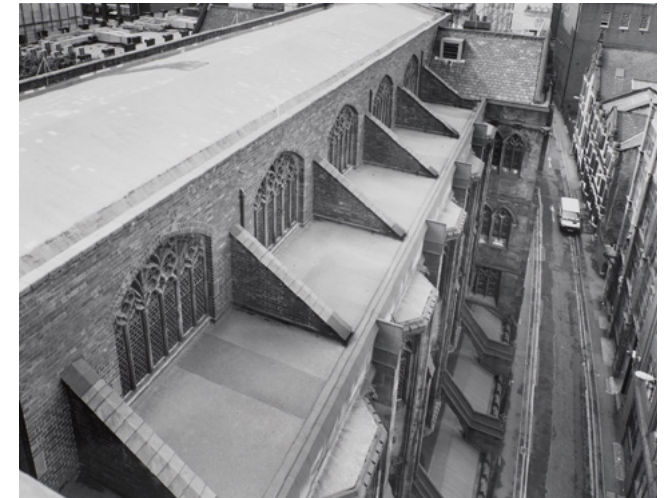
2.9 South clerestory and cloister roof, 2003 (UoM)
