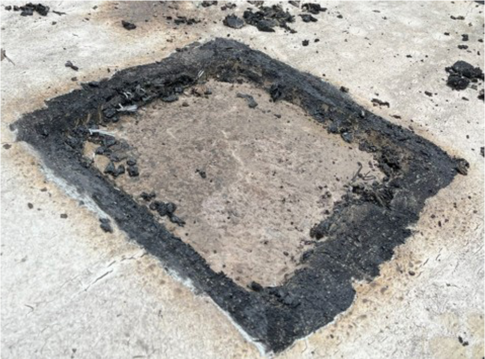
3.11 Opening Up Works
