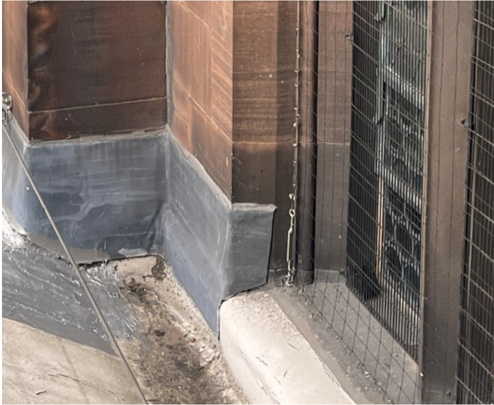
3.8 Asphalt Gutter, Asphalt Sill, Lapped Lead
