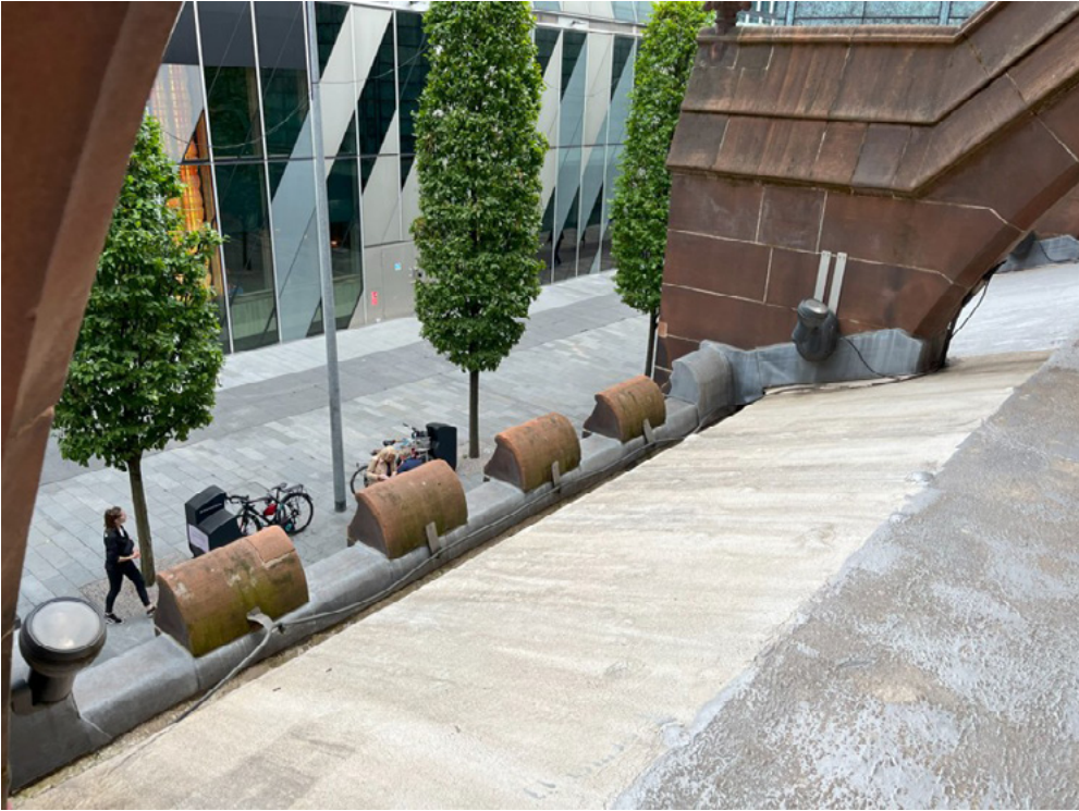
3.3 Brazenose Street Cloister Roofs
