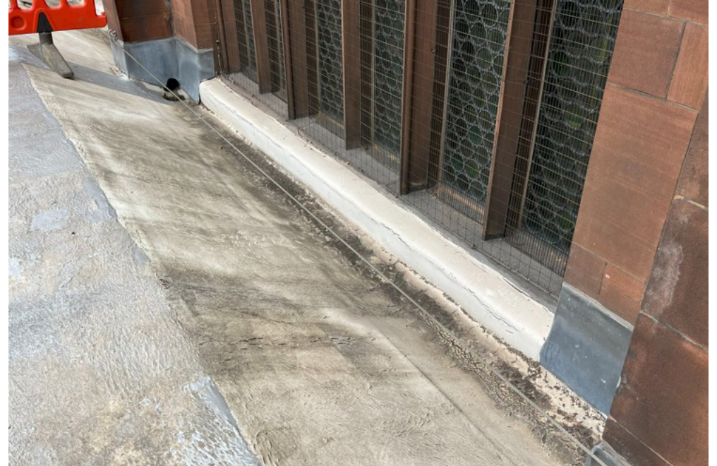
3.7 Asphalt Gutter, Asphalt Sill, Lapped Lead
