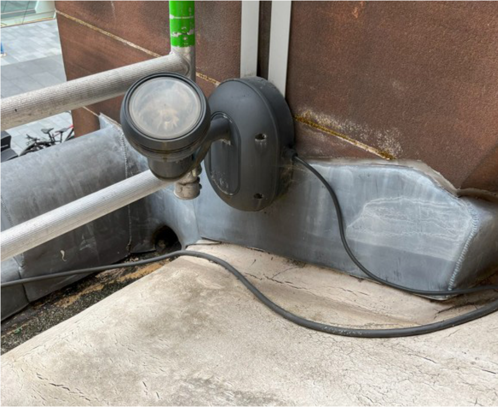
3.9 Asphalt Gutter with Buttress Passthrough
