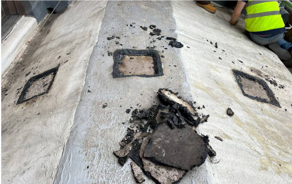
3.10 Opening Up Works
