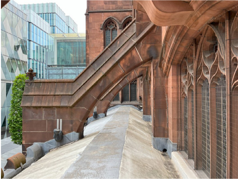
3.2 Brazenose Street Cloister Roofs
