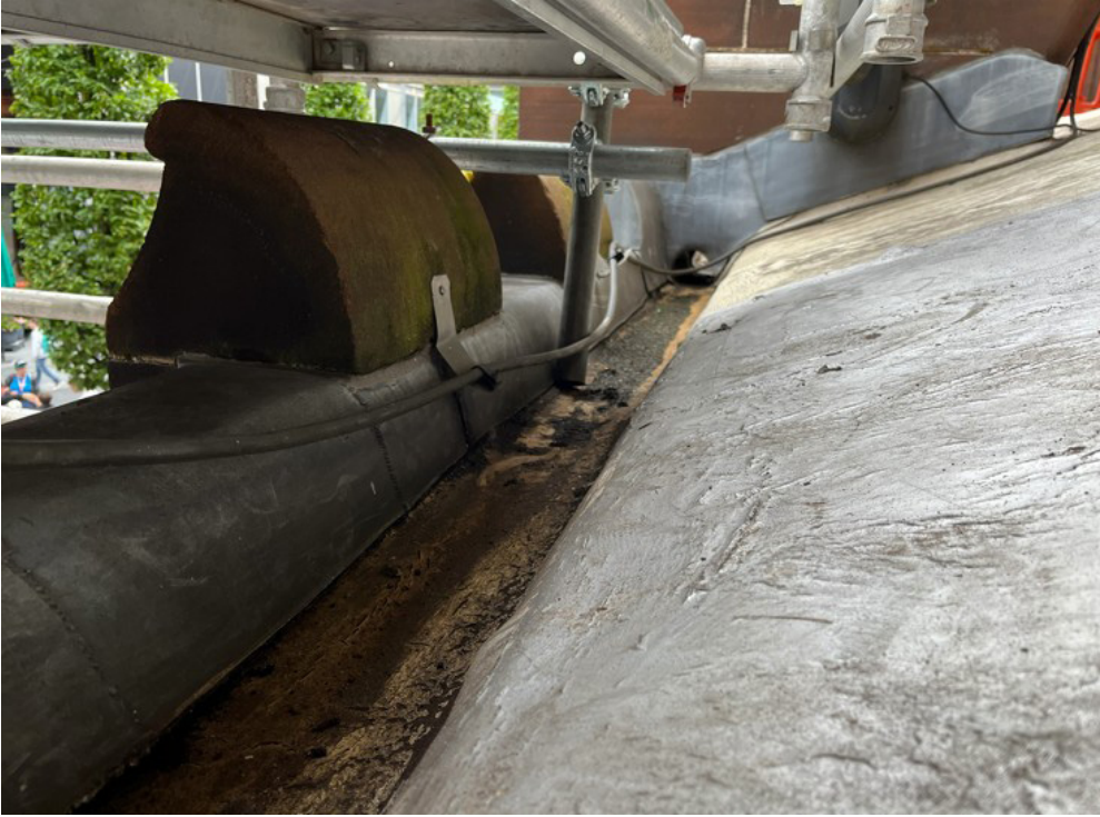
3.5 Asphalt Gutter with Lapped Lead
