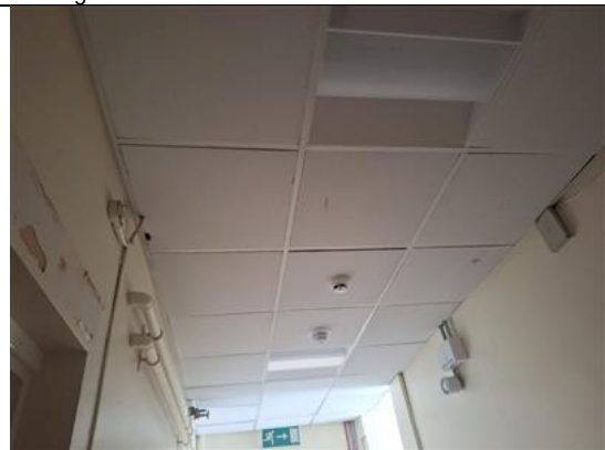
Photo 10 (08/07/2025): Internal view of room within the south, eastern section of the building.
