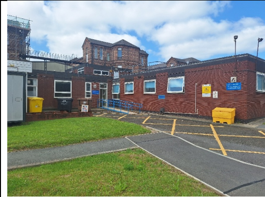
Photo 1 (08/07/2025): Northern and eastern aspects of the building.
