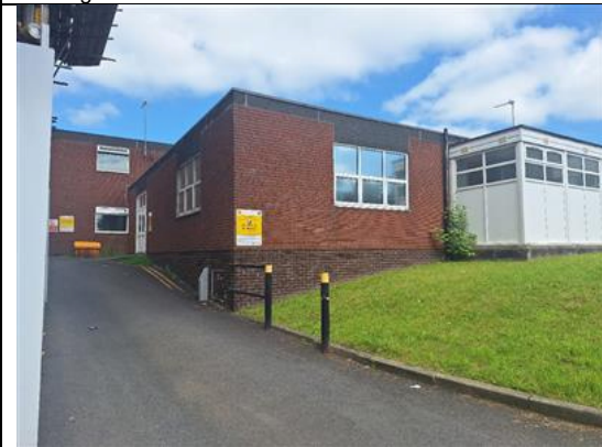
Photo 3 (08/07/2025): Southern and eastern aspects of the building.
