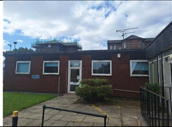
Photo 8 (08/07/2025): Northern and eastern aspect of the building.
