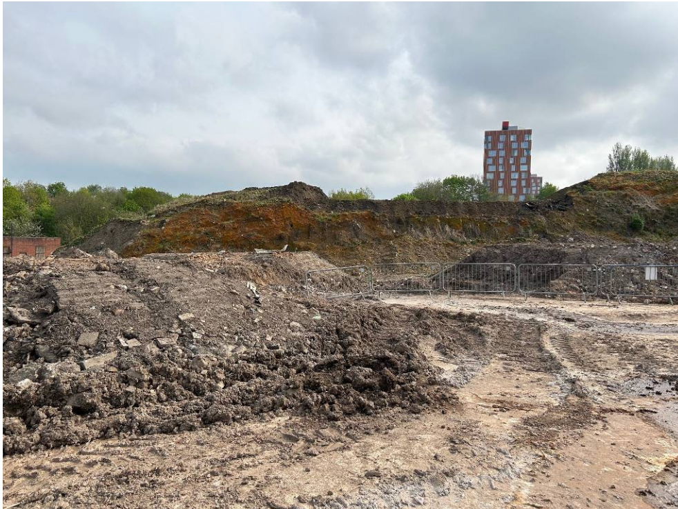
Stockpiles of material on Plot NT03 and NT04
