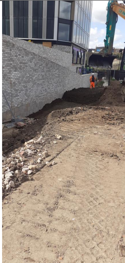
Backfilling to boundary wall – NT02
