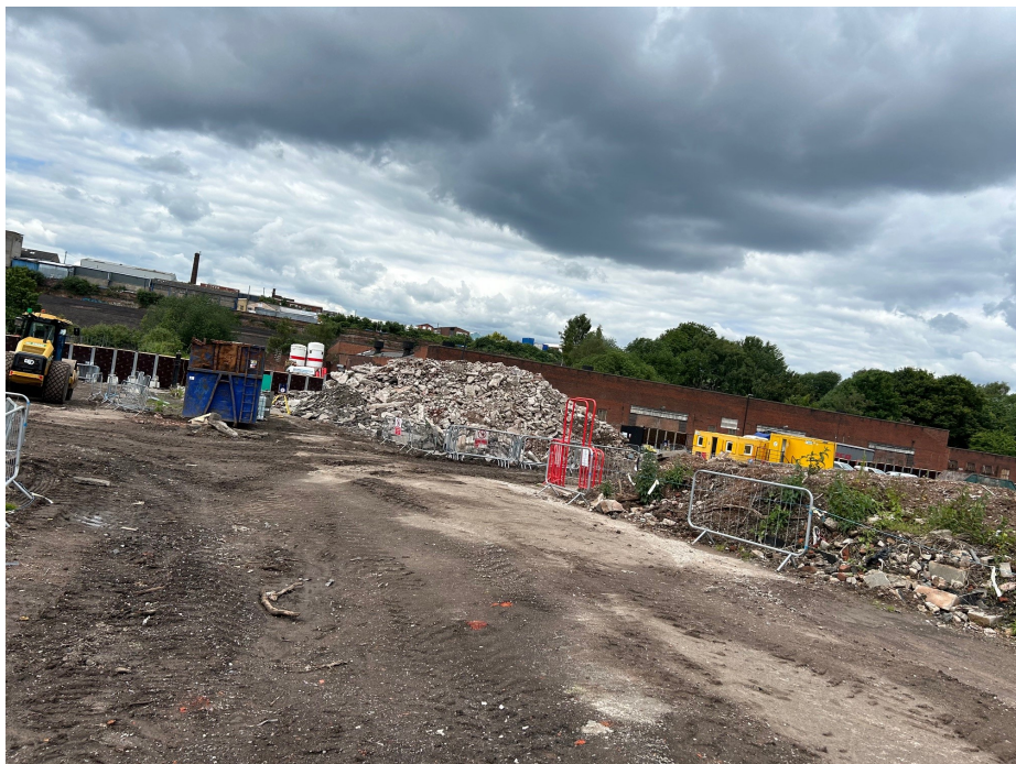
NT02 Slab broken out and surface compacted
