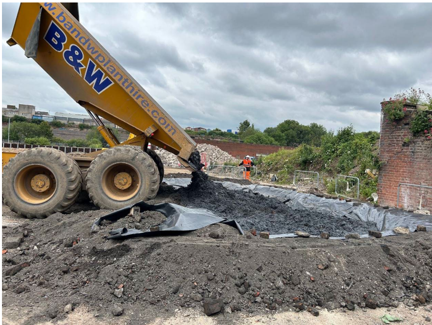
LFT01 Tank Storage bund for excavated material
