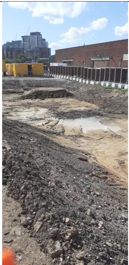
Excavated area within NT04 – minor ponding of water
