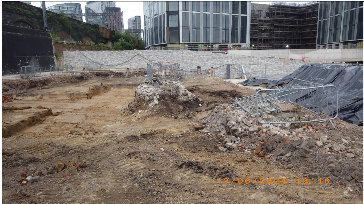
Facing west in TCE area.
