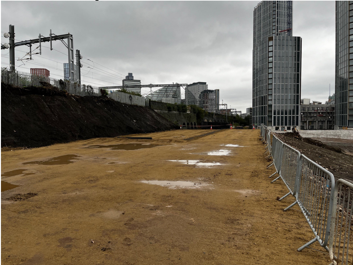
Network Rail Mound Piling Platform
