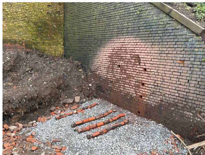
Network Rail eastern wing wall cores
