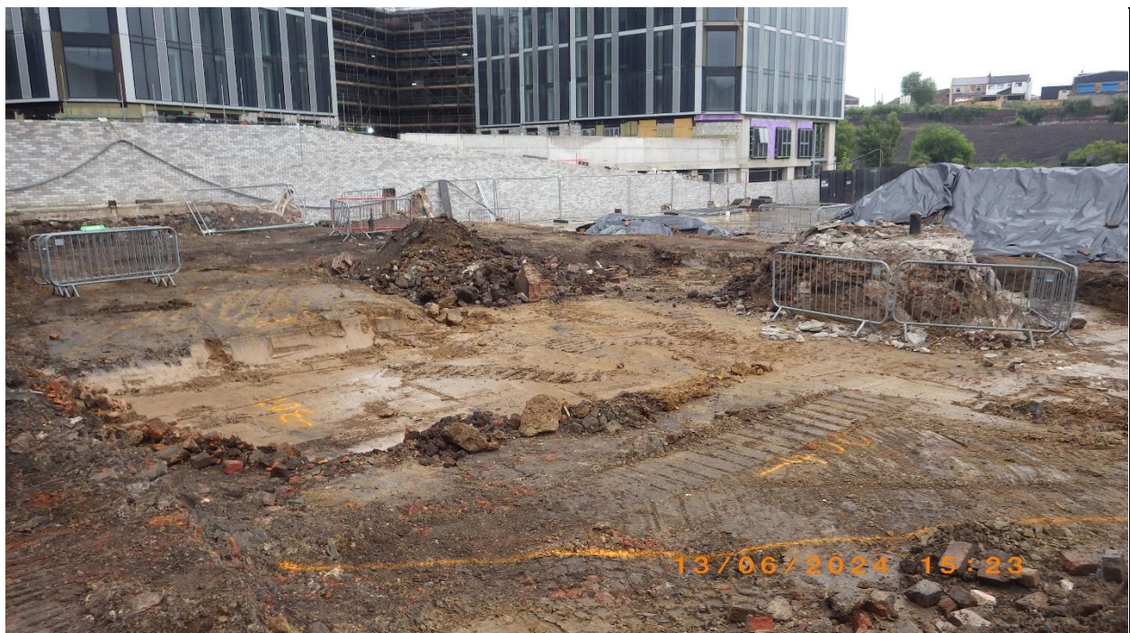
Facing north west in TCE area during first round of excavations
