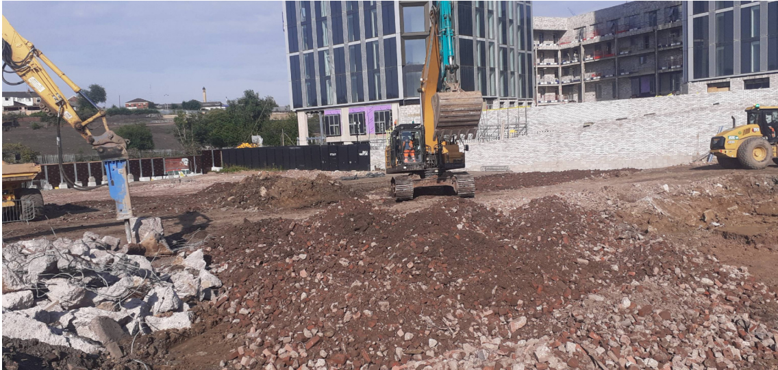
NT02 Storage tanks removed, relic foundations removed and ongoing earthworks
