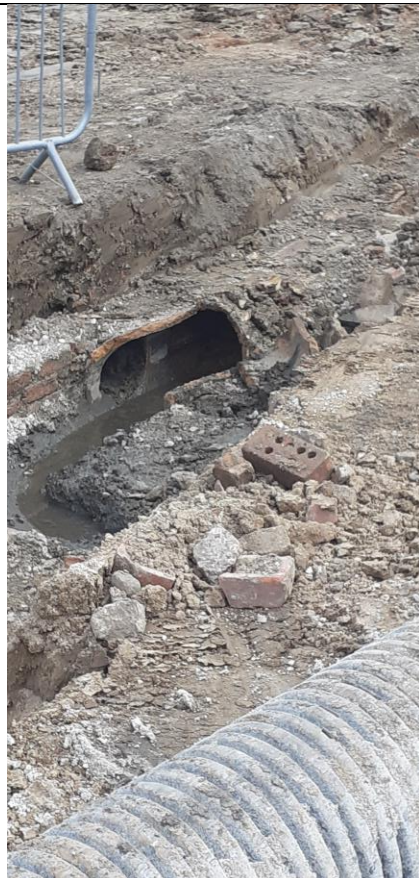
375mm dia SW pipe – note lateral pipe connection
