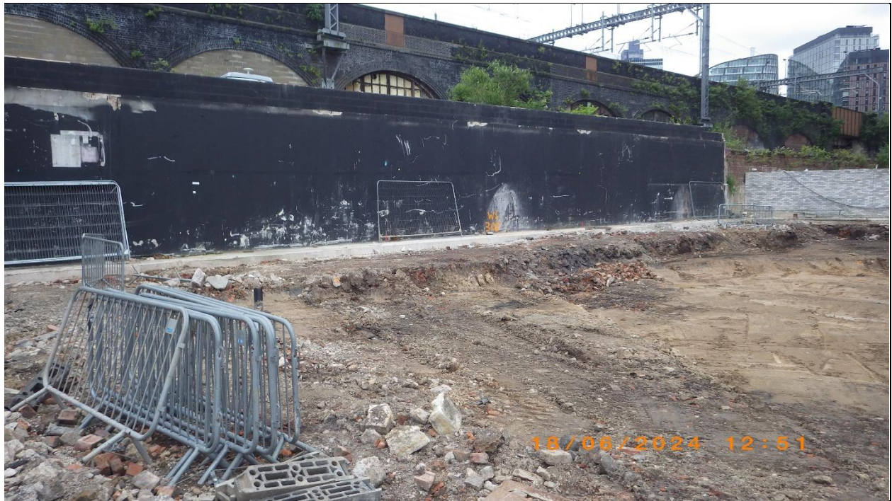
Facing south, note standoff from garage retaining wall
