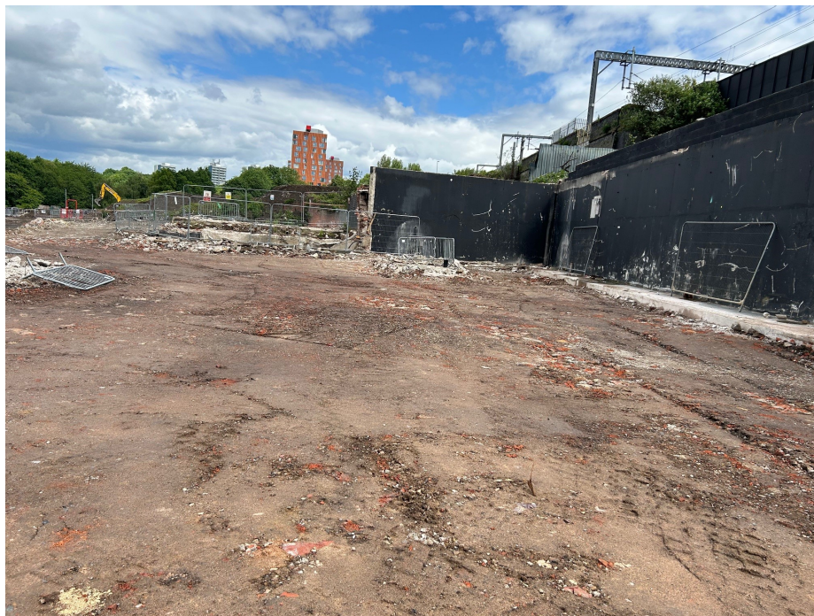
NT02 Slab broken out and surface compacted
