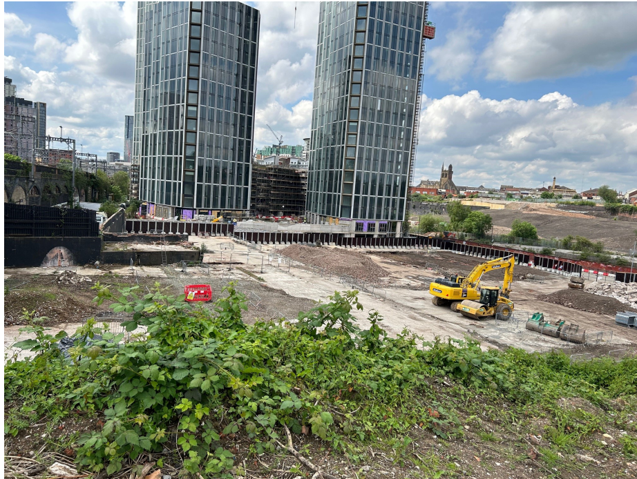
Stockpiles of material on plot NT03
