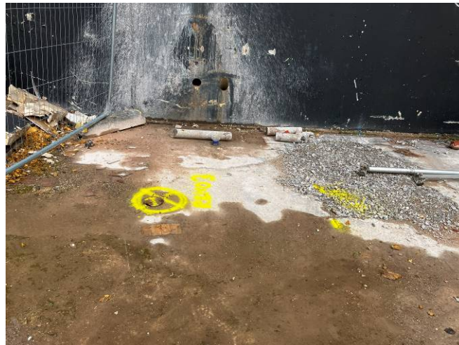
Network Rail eastern wing wall cores
