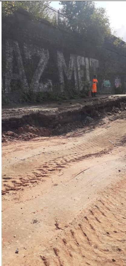
Ramp to piling platform progressing NT04 – can ground be battered along retaining wall?
