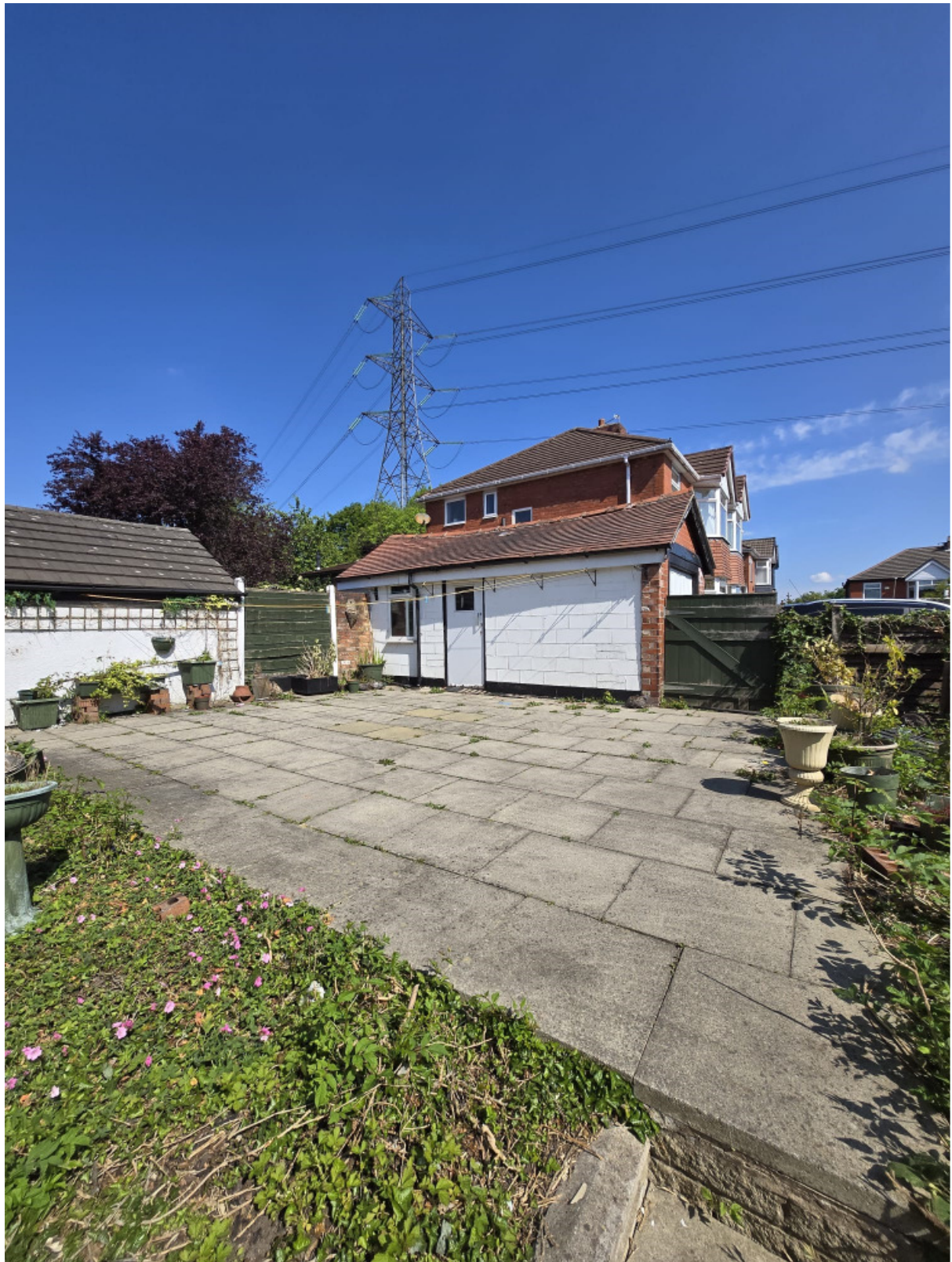
Above original garage used as second kitchen – note waterpipes to gully from sink below window
