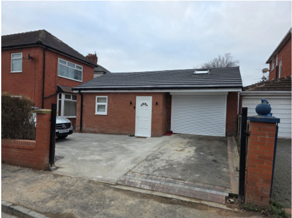
Above : completed outbuilding
