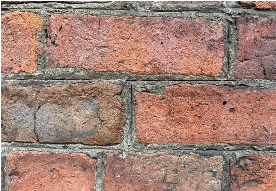
Figure 22: A detailed view of the surviving original c1830s pointing to the north-east corner of the building, which can be seen to have “penny” pointing.
