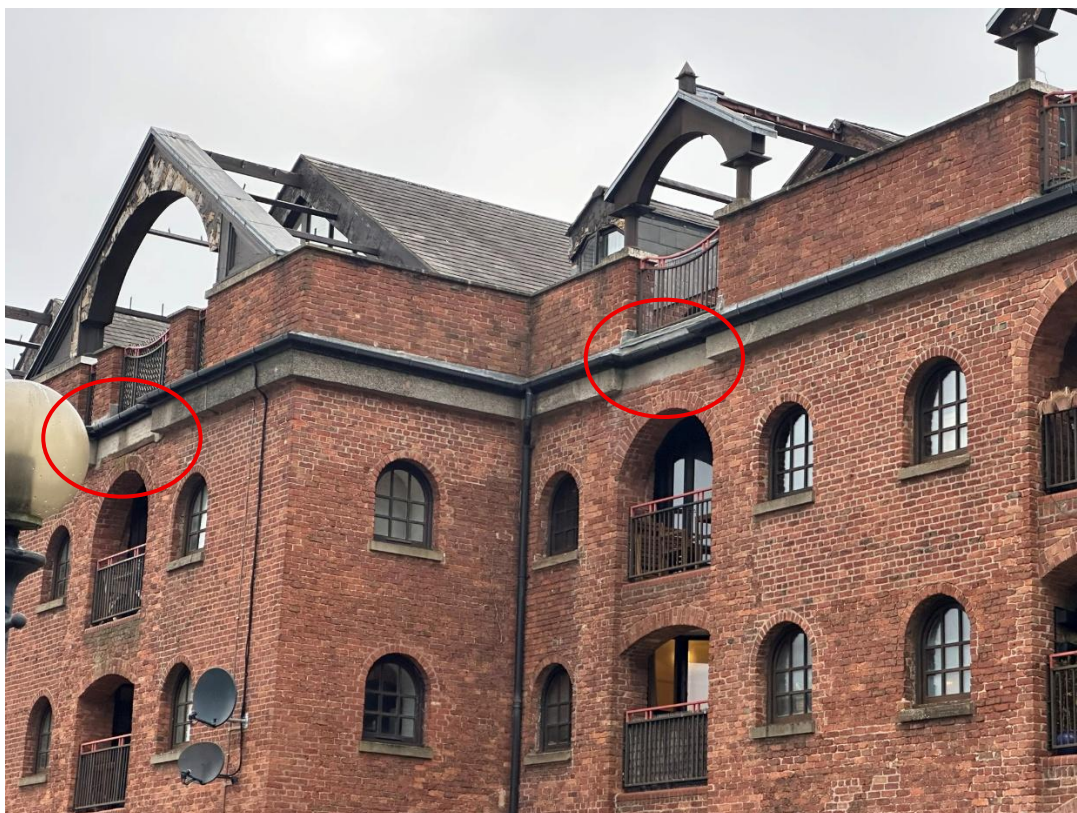
Figure 18: A view looking up at the upper part of the south elevation, illustrating the c1920s reinforced concrete ring beam and modern parapet brickwork.
