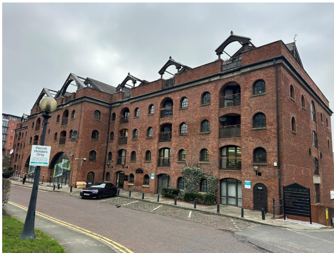
Figure 17: A view looking north-west towards the south (left) and east (right) elevations from Castle Quay, illustrating three of the six original “loopholes” which were extended with reinforced concrete structures in the c1920s and demolished as part of the 1980s works.
