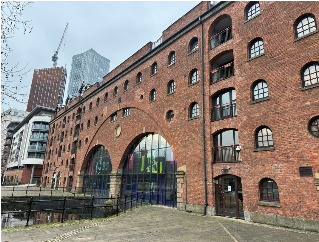
Figure 23: A view looking across the north elevation from the western side of the basin.
