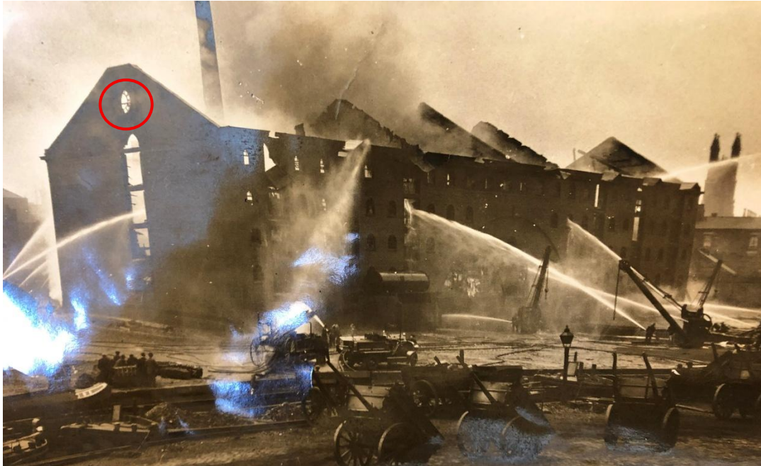
Figure 8: 1A view looking south-west towards the north and east elevations of Middle Warehouse from the basin showing the fire that destroyed the majority of the building in 1919.
