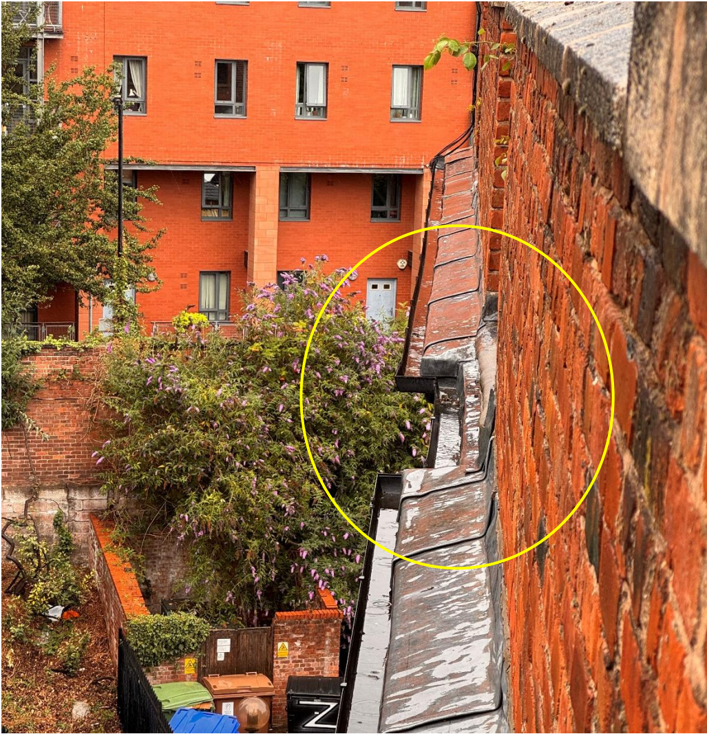
Figure 25: A view looking west along the parapet of the building, illustrating the inherent design flaw from the 1980s development, which saw new leadwork and guttering being installed to follow the recesses within the 1920s concrete ring beam in five locations along the south elevation – which has resulted in an inadequate rainwater run-off from the top floor apartment balconies causing long-standing water ingress issues for residents.
