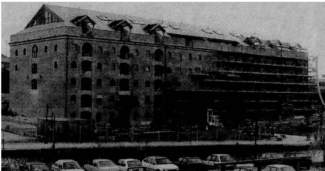
Figure 13: A view looking south of the conversion of Middle Warehouse nearing completion.
