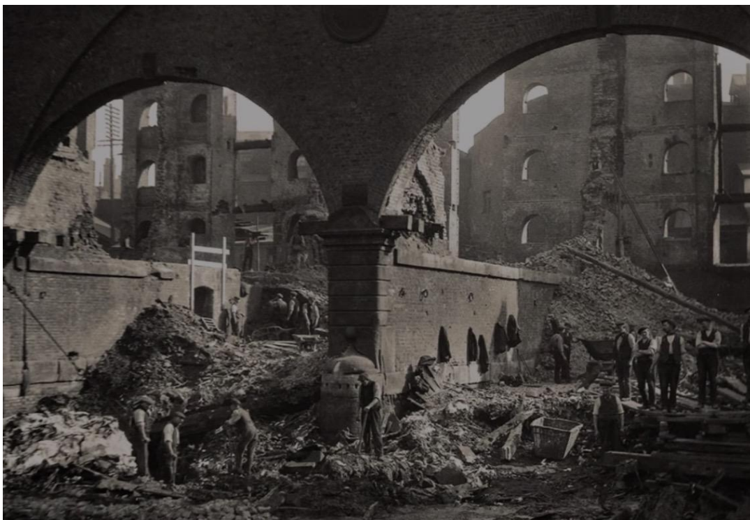
Figure 9a: A view looking into the northern boat holes in the days following the 1919 fire, showing the total destruction of the interior of the warehouse.
