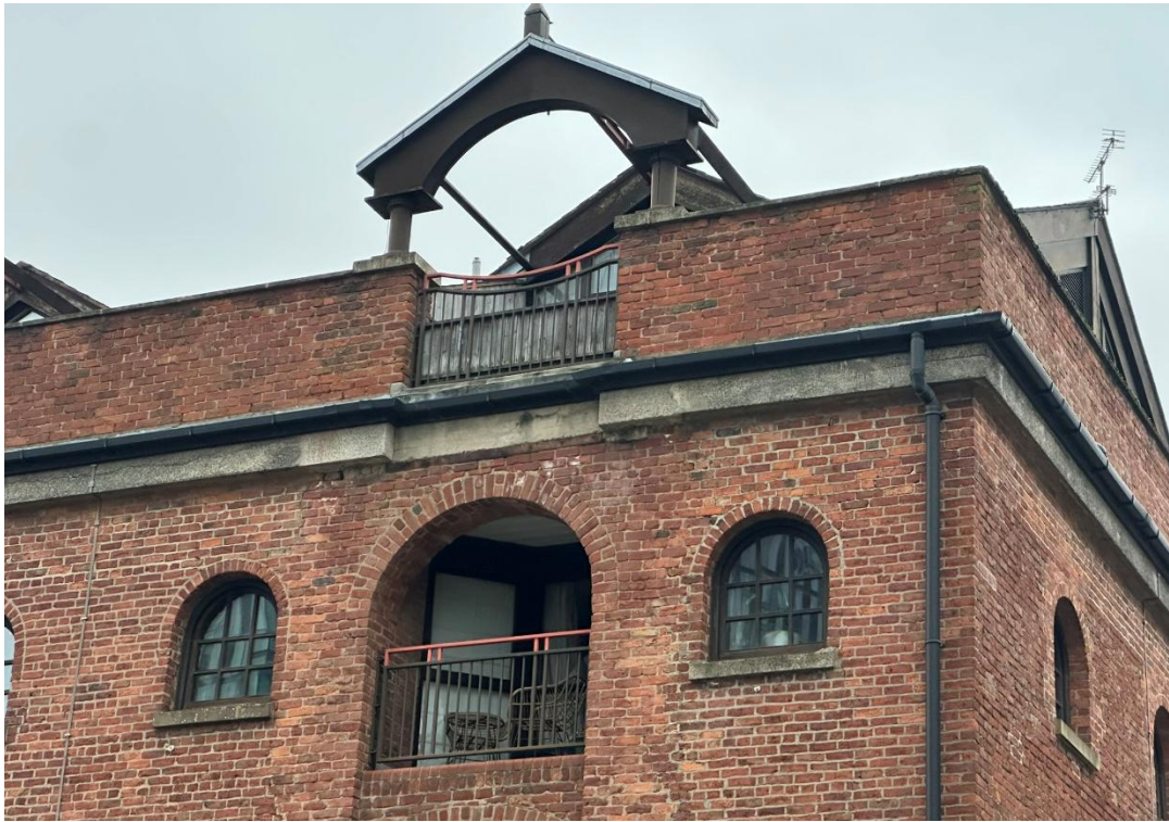
Figure 19: A Looking up at the south-east corner, showing the concrete ring beam and recess from the now demolished 1920s extension.
