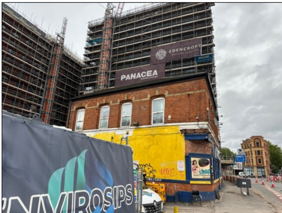
Photograph 4, A view of the western face of the building. The western side is to face the proposed apartment block. Again, small openings on the first storey exterior were hollow when assessed with binoculars.
