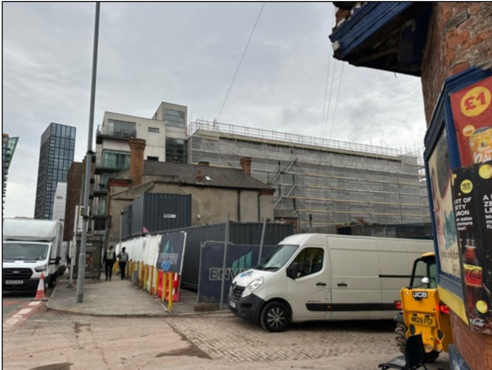
Photograph 7, A view of the land on site, which features west of the building. This is exclusively hard standing and features a welfare unit atop for the nearby development works. This plot is to accommodate the proposed apartment block.
