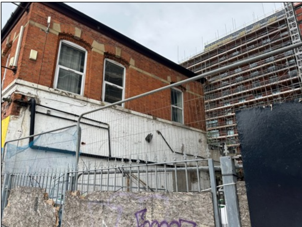
Photograph 2, A view of the fencing along Rochdale Road footpath, which borders the site.
