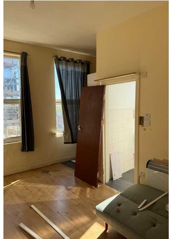
Photograph 11; A photograph of a previous internal survey of the building, showing a section of previous dwelling space.
