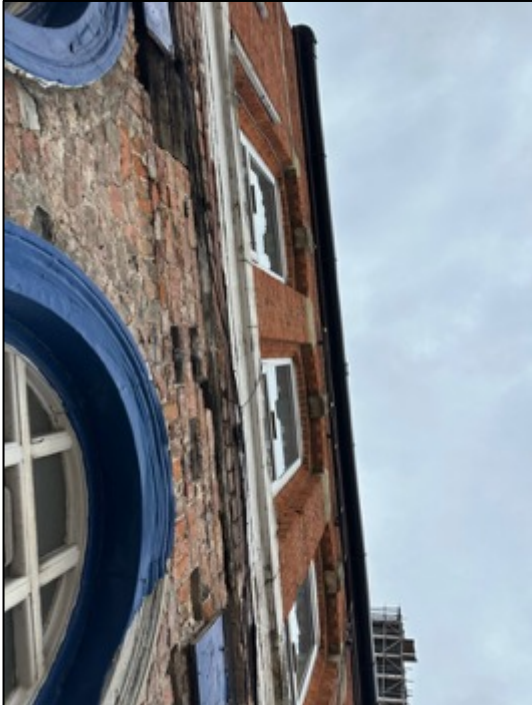
Photograph 10; A view of the front of building, showing the various entry points across the first storey face. Again, these openings were hollow and mostly 1 brick/half-brick deep and likely created by alterations and previous exterior fittings.
