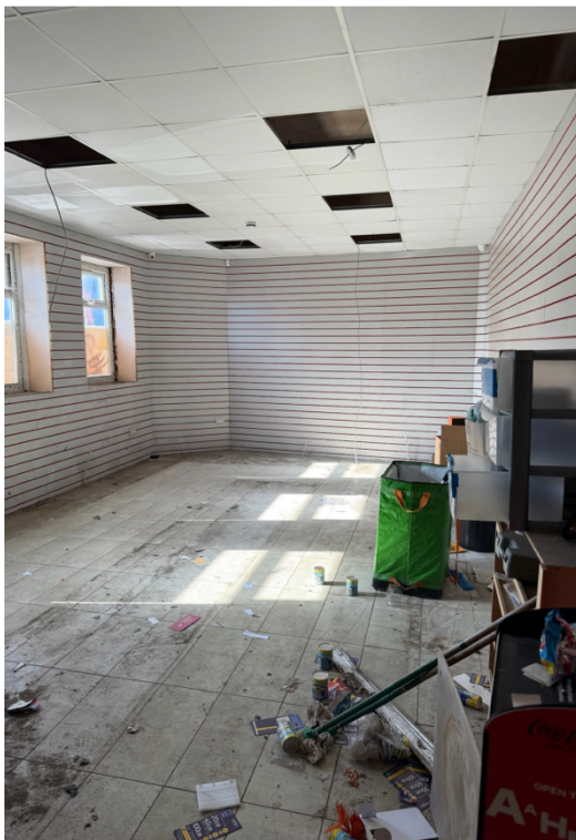
Photograph 12; Another photograph of previous internal survey. Some sections of the upper floor feature suspended ceiling.
