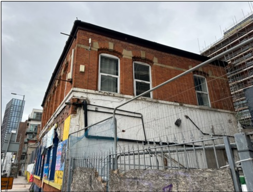
Photograph 1, A view of the eastern face of the building on site to be retained. The building is traditional brick, with a single storey mixed painted face. Some slight displacement was noted across some brick decal points above windows.
