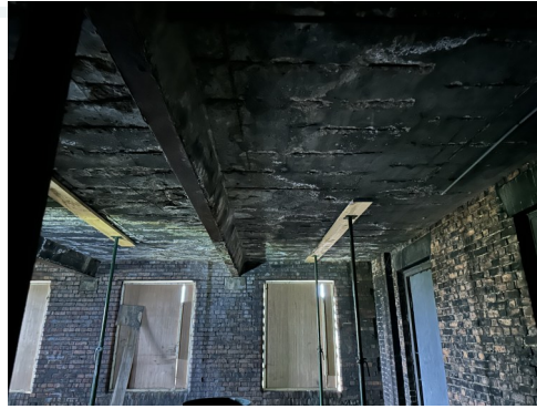
Photo 2 - Waste House Roof
