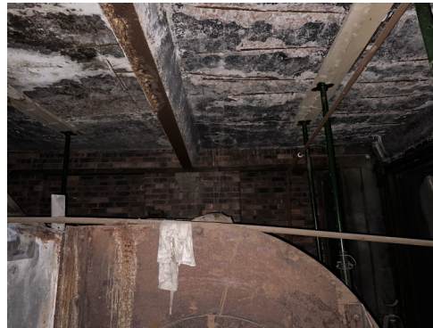
Photo 6 - Waste House Roof
