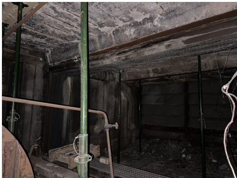
Photo 5 - Waste House Roof
