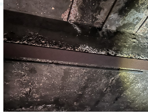
Photo 3 - Waste House Roof
