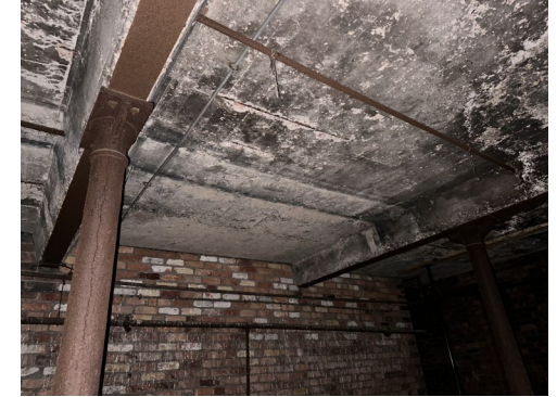
Photo 4 - Waste House Roof
