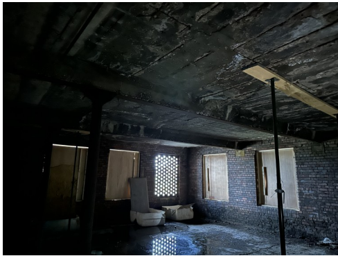
Photo 1 - Waste House Roof
