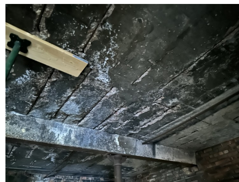
Photo 7 - Waste House Roof
