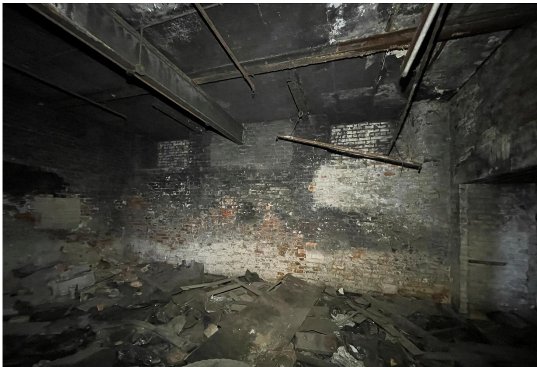
Figure 16 – A view looking towards the south-east (rear) wall showing the three blocked windows which would have looked onto the canal.
