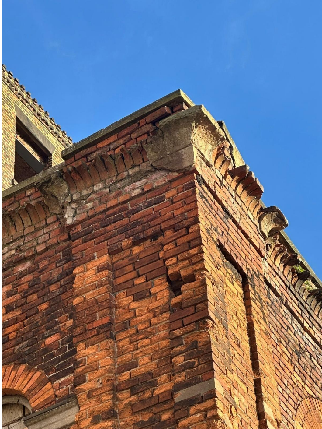
Figure 13 – Detail of the northern corner of the engine house, illustrating the original brick and stucco arrangement.
