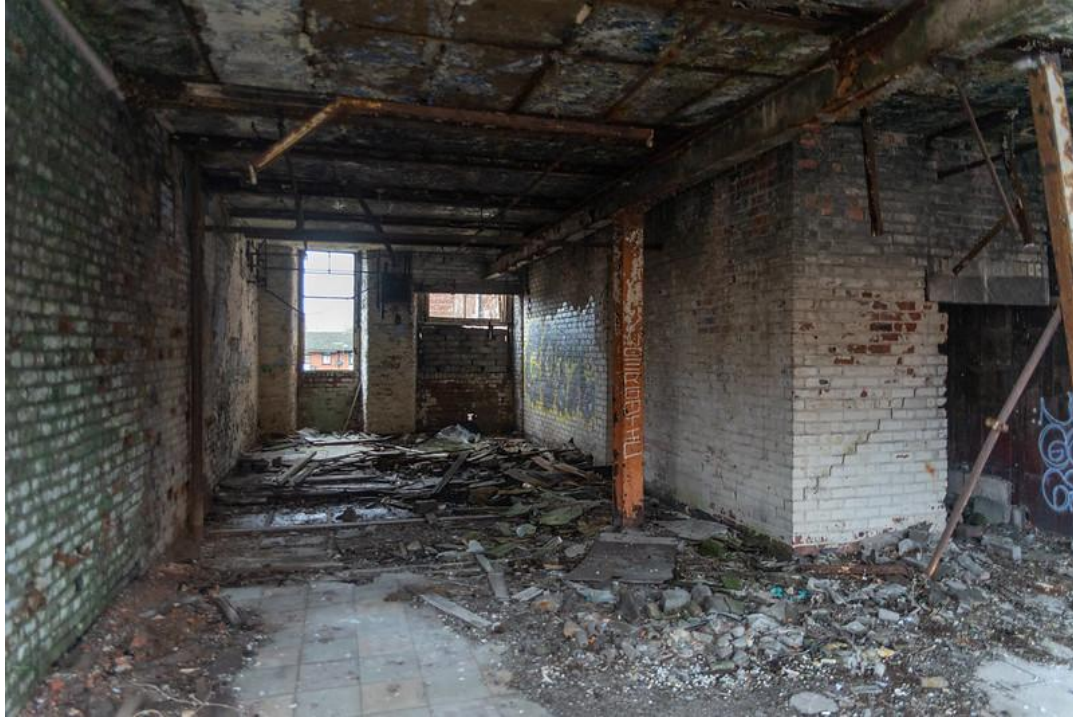
Figure 18 – A view looking north across the first floor level, which was formed with the c1950s reinforced concrete floor and ceiling.
