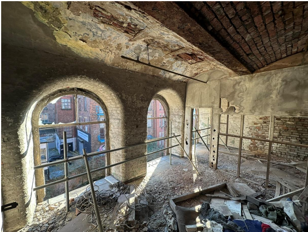
Figure 21 – A closer view of the southern three windows, showing their deep reveals and bullnose edges. Note the original brick, jack-arched ceiling/roof.
