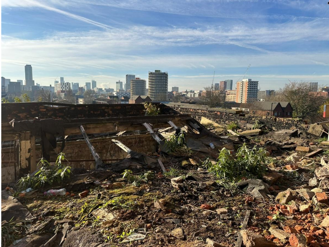
Figure 14 – A view looking west across the engine house roof, showing the raised timber skylight to the centre of the flat roof.
