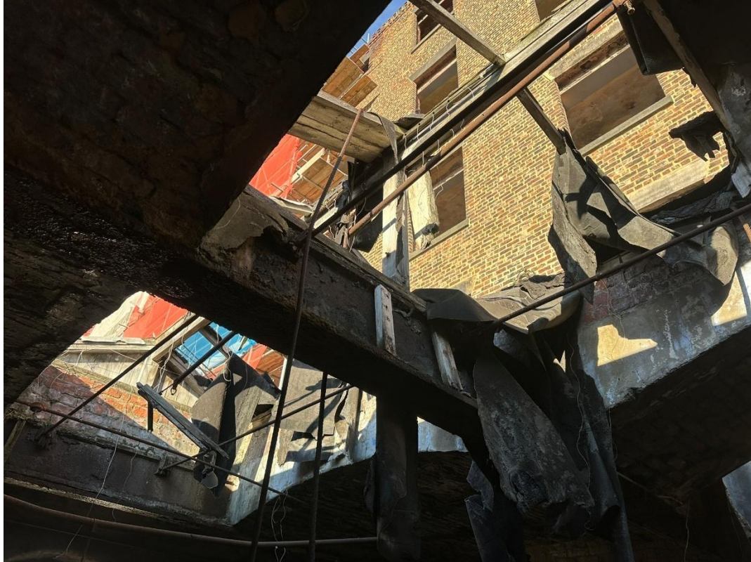
Figure 27 – Looking up at the original central skylight and the remains of its timber skylight structure.
