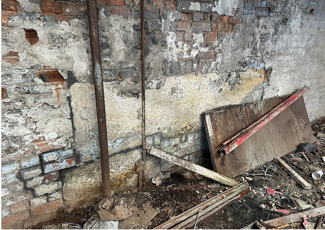
Figure 25 – A view of the original stone bearing blocks to the north-west wall from which would have supported the original flywheel of the steam engine.
