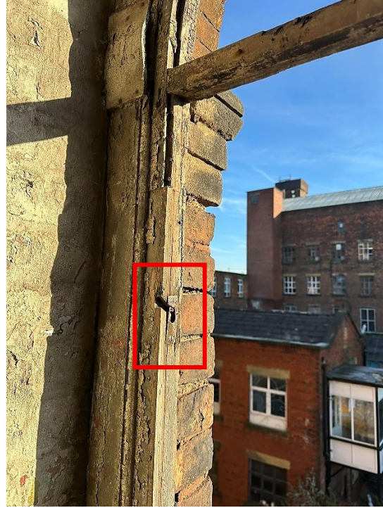
Figure 23 – A detailed view of one of the southern windows showing evidence of original opening fixings to the frame.
