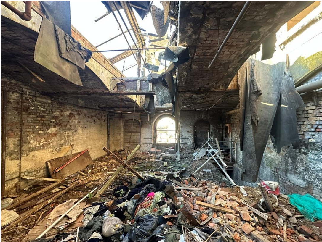
Figure 19 – Looking north across the top, second floor level, formed in the c1950s with the insertion of its concrete floor, which runs across all window openings.
