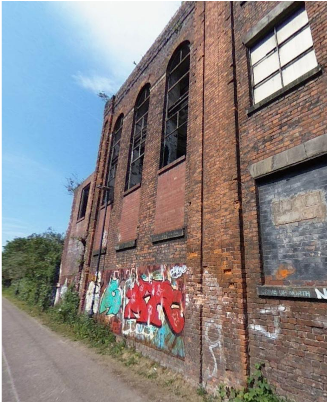
Figure 12 – A view of the rear, south-east elevation as seen from the canal towpath, showing the three original window openings.
