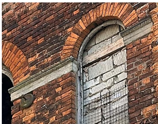
Figure's 7 & 8 – A view of the principal, northwest elevation, showing one of the three round-headed window openings with carved stone (possibly grit stone) string course between the windows (Figure 7) and a view of the stringcourse from inside the building (Figure 8).
