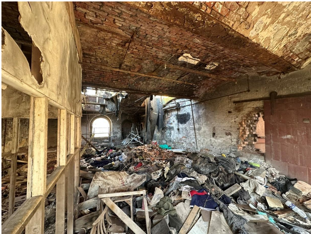
Figure 24 –A view looking north across the second floor level.
