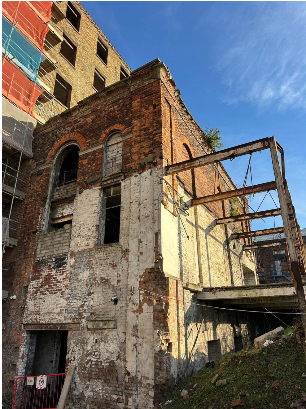
Figure 11 – A view looking towards the north-west elevation (left) and south-west elevation (right) which illustrates its three original blind openings.
