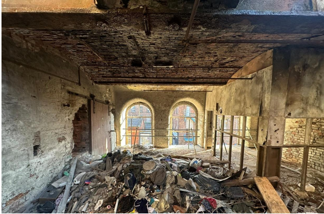
Figure 20 – Looking south towards the rear elevation, showing the three original round-headed window openings onto the canal.
