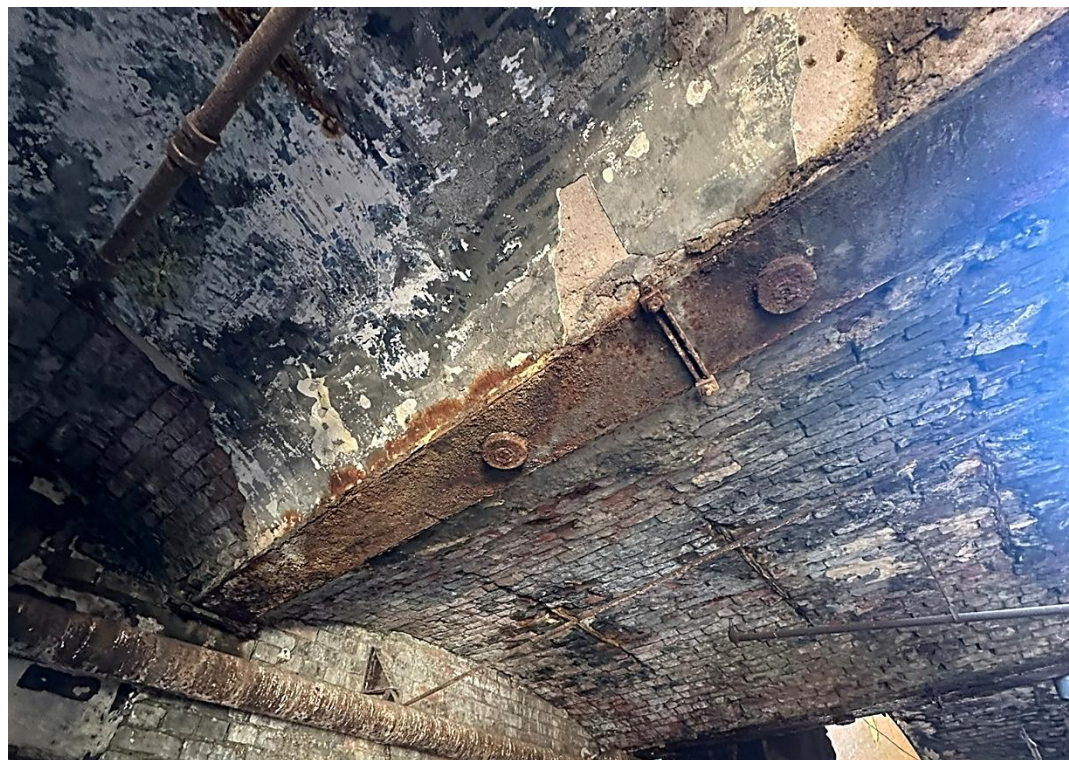
Figure 28 – Detailed view of the original jack-arched ceiling.
