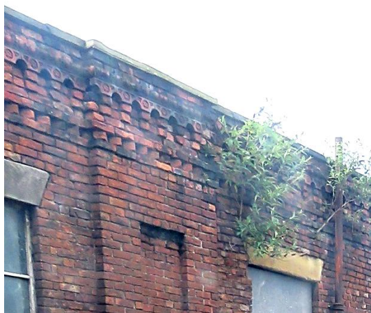
Figure 5 – An example of the c1880s/90s replacement of the original stuccoed eaves detailing with moulded, decorative redbrick as seen around the perimeter of the main mill.
