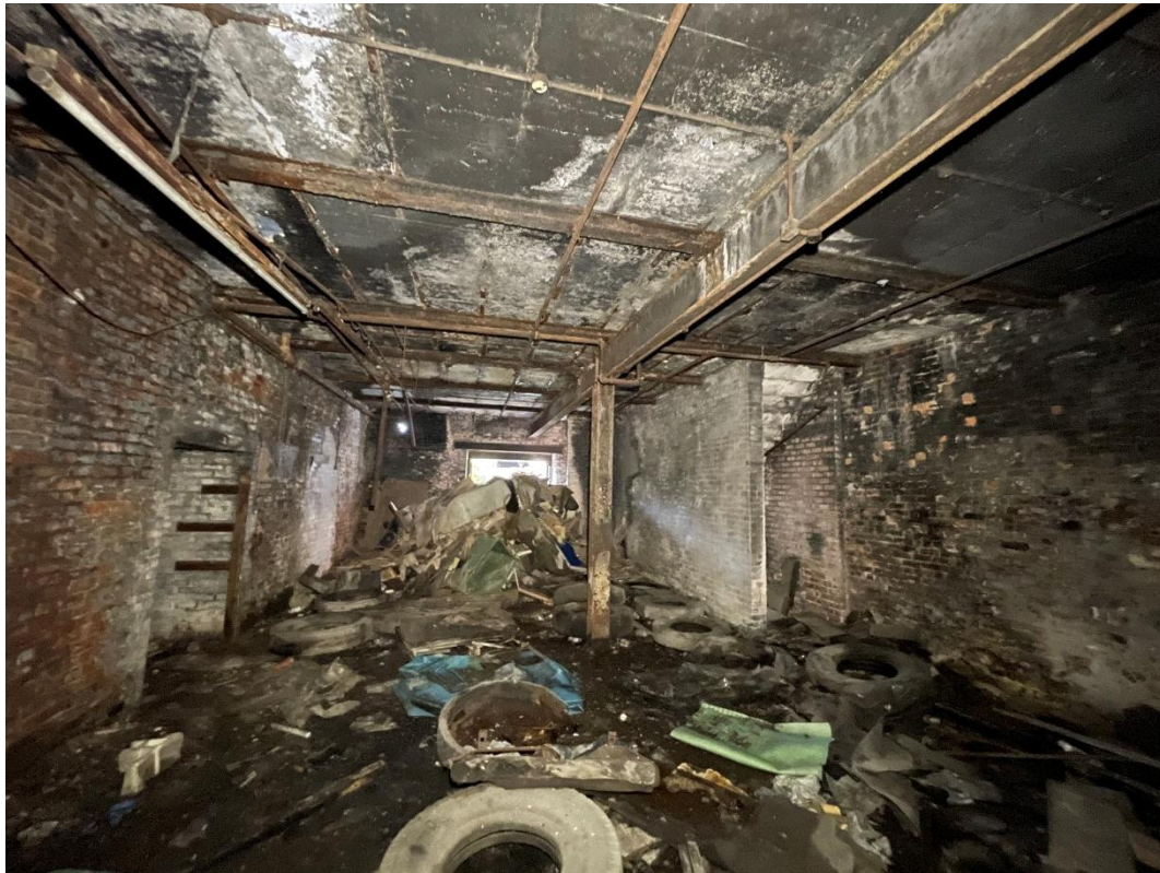
Figure 15 – A view looking north across the ground floor level, showing the inserted c1950s concrete floor and staircase (left) at a slightly higher level.
