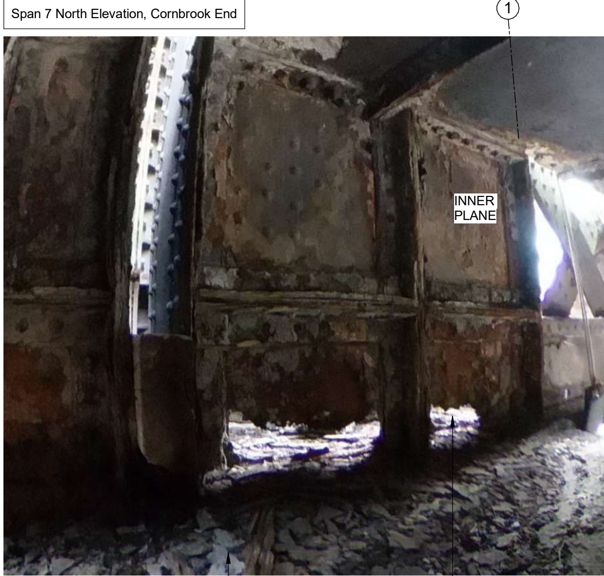
Span 7 North Elevation, Cornbrook End Debris at pier head to be cleared to confirm extents/condition of bottom horizontal stiffener on GL A Holes on both lower web panels, inner plane
