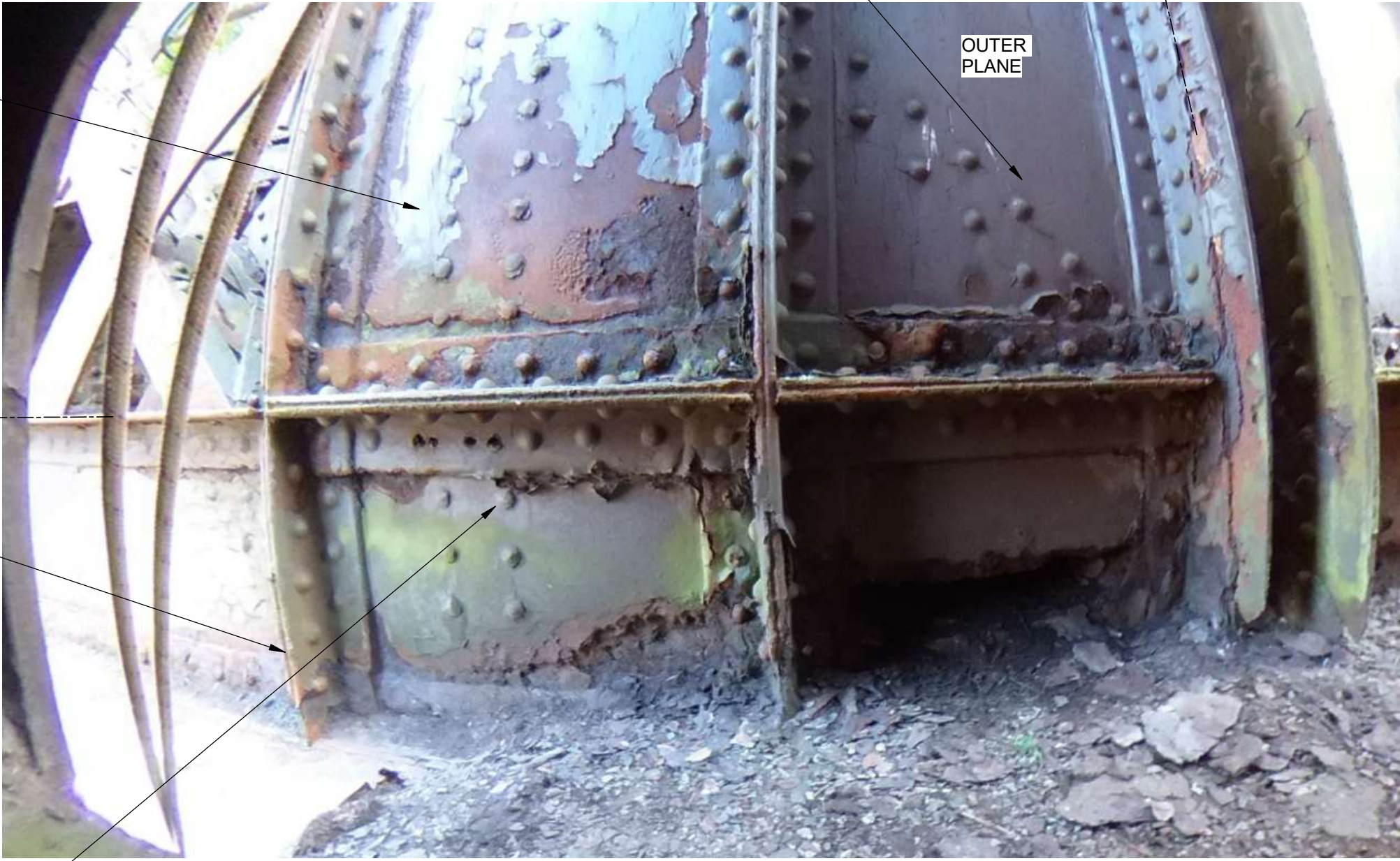
Span 4 South Elevation, Cornbrook End
