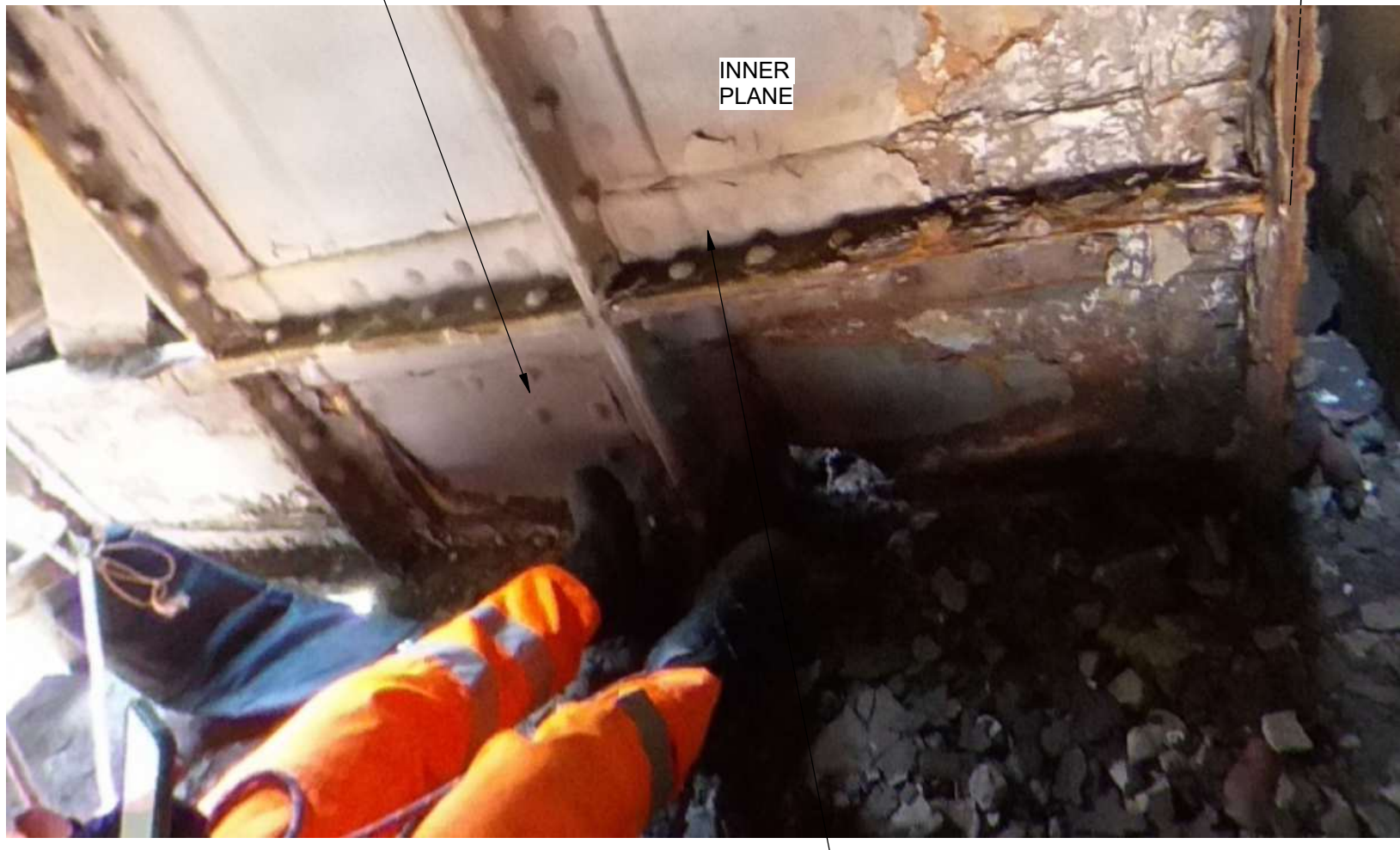
Span 4 South Elevation, Cornbrook End
