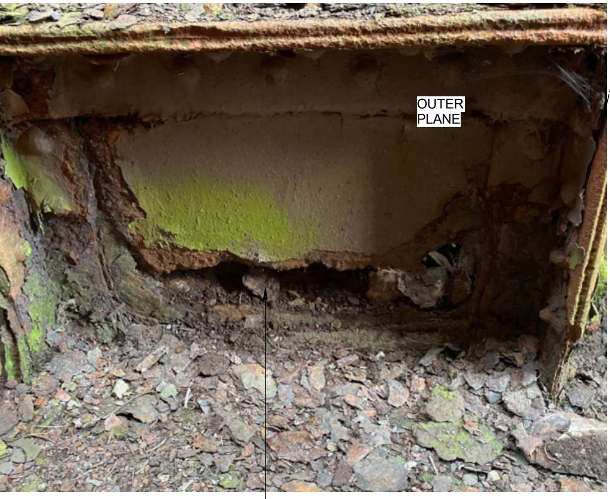
Span 4 South Elevation, Cornbrook End
