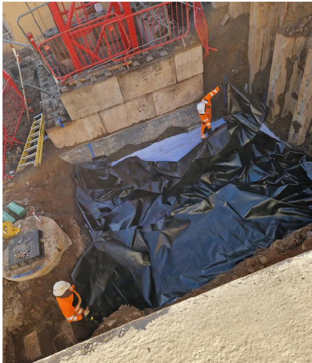
Figure 1: Impermeable Membrane Placed at Base
