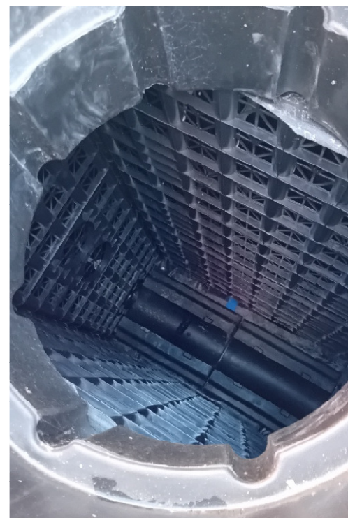
Figure 4: Access into Tank for Maintenance
