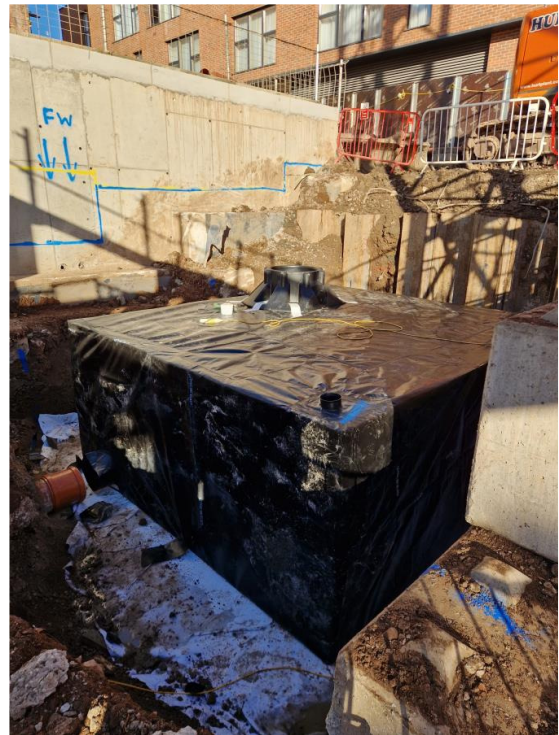
Figure 2: Geocellular Crates wrapped in Membrane
