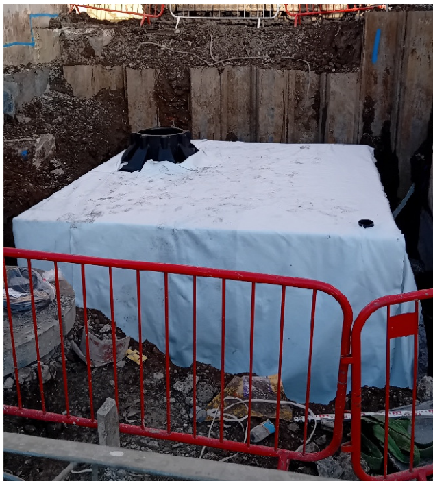
Figure 3: Tank wrapped in Fleece Protection
