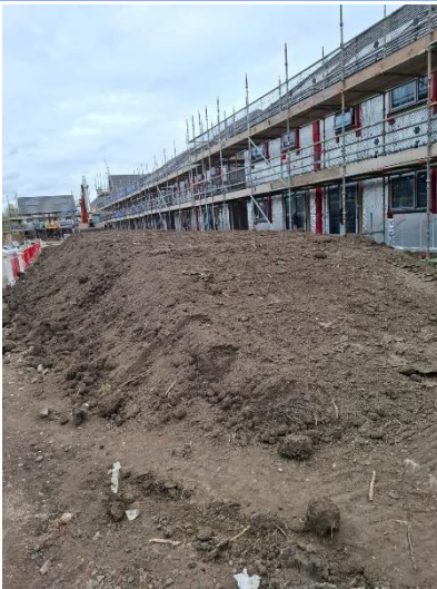
Photograph 1 – Front view (looking east)
