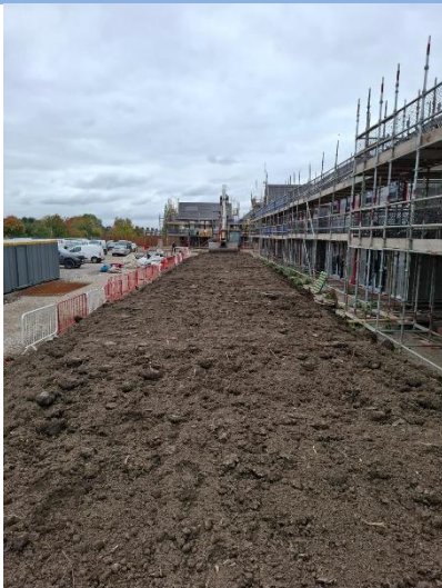
Photograph 3 – Top of SP
