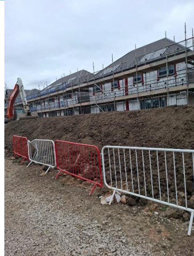
Photograph 2 – Side view (looking south)
