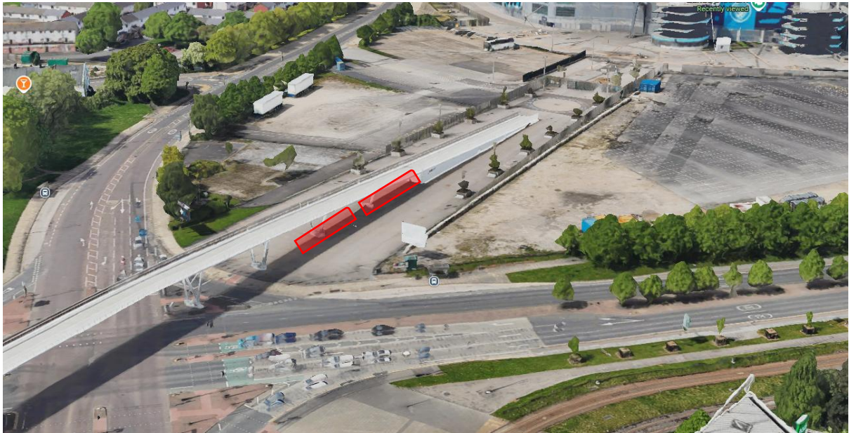
Image 3: Red indicates location 2 under the footbridge
