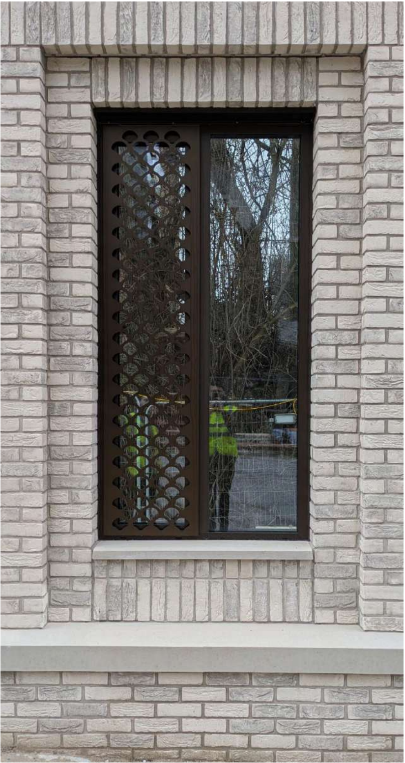
3 - Brickwork Typical Bay
