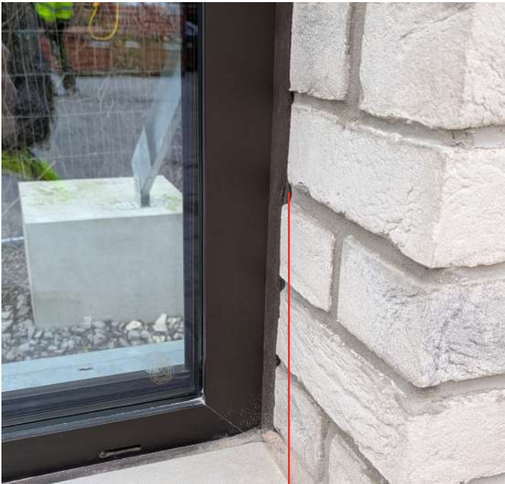
2. Mastic Spilling
